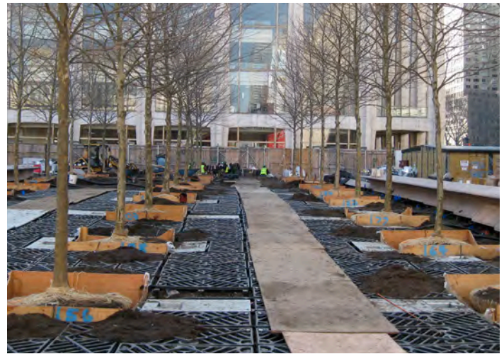
Soil cell installation at Lincoln Center New York (image: DeepRoot, CC BY-NC-ND 2.0, Flickr)
