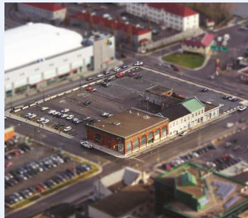
Block 4: Existing Condition
