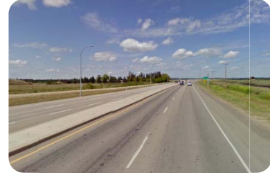
Paved shoulder on a multi-lane rural highway, AB (Google Streetview)
