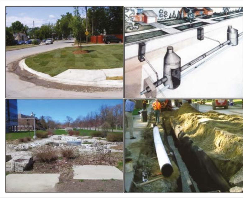
Example LID Practices from Top Left to Right: Soil Amendment (Mississauga, ON), Exfiltration System (Etobicoke ON); Exfiltration System (Guelph, ON); Perforated Pipe (Toronto, ON)
