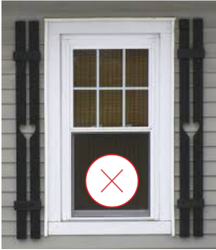
63. Incorrectly proportioned new shutters. (Source: oldhouseguy.com)
