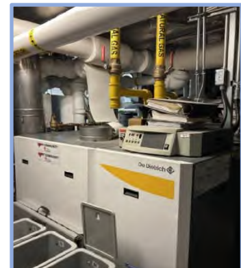
Central Heating Boilers
