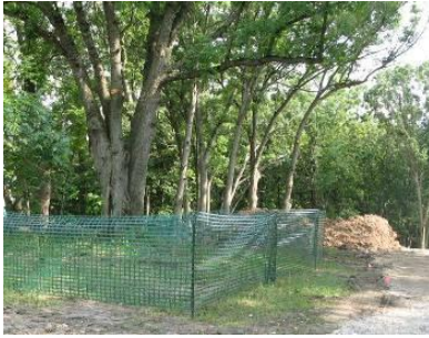
Trees identified for retention are protected by barriers during construction
