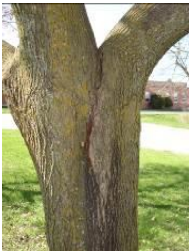
Lack of regular inspection and timely pruning leads to premature tree failure, and unnecessary loss of public assets.
