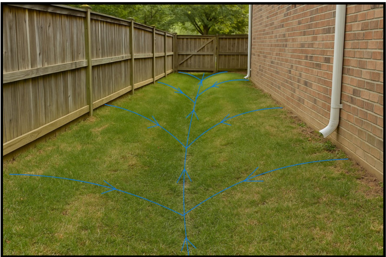
IMAGE 1: SIDE YARD SWALE
