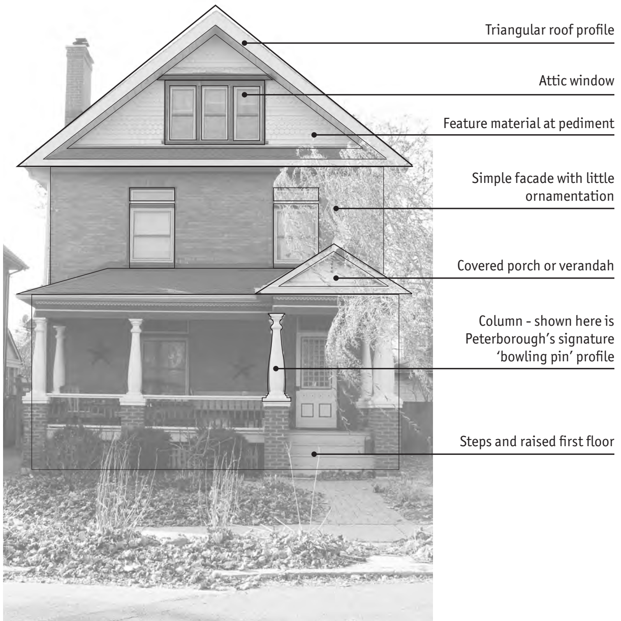
43. Diagram showing some key features of Edwardian front gable houses. Source: ERA 2013.
