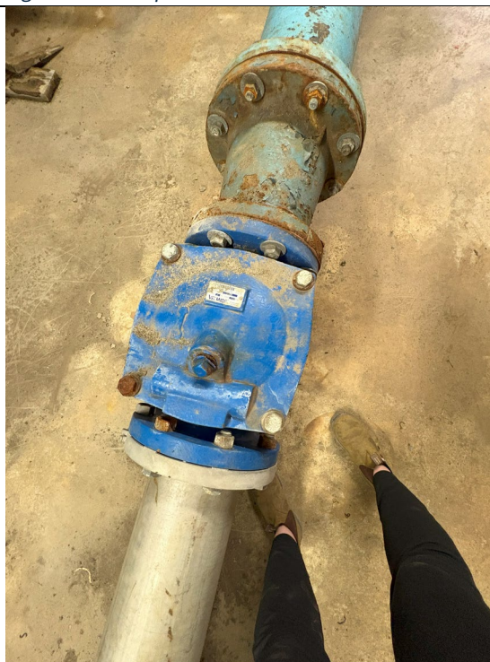
Figure 154: Swing Check Valve on Pump #2
