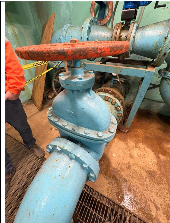
Figure 567: Zone 1 Feed Gate Valve
