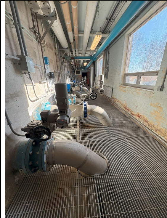
Figure 55: Drain Actuator on Filters 7, 8 & 9
