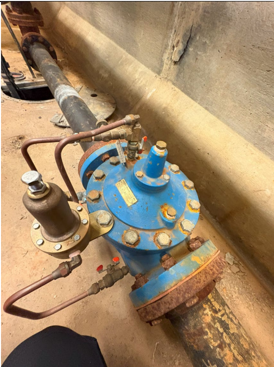
Figure 322: 6" Pressure Reducing Valve
