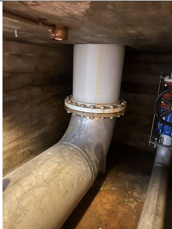
Figure 444: 500mm Stainless Steel Piping, Tower Intake
