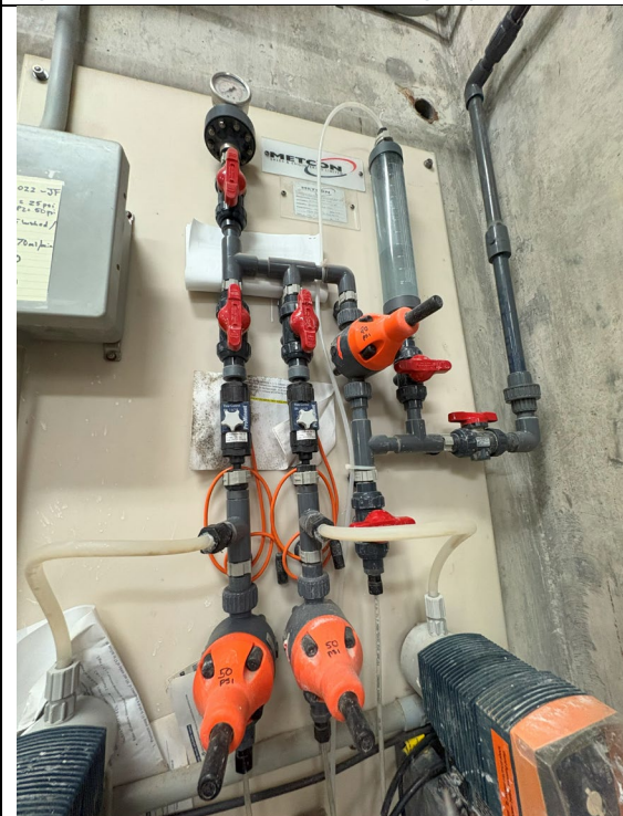
Figure 135: Dechlorination Controls
