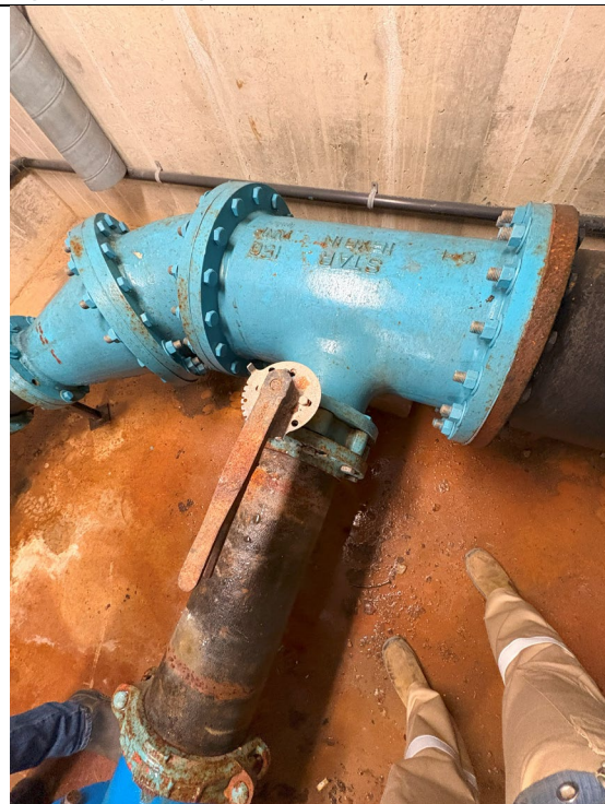
Figure 190: Butterfly Valve on Pump #2
