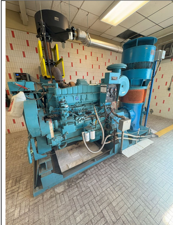
Figure 61: Pump #1 Diesel Motor
