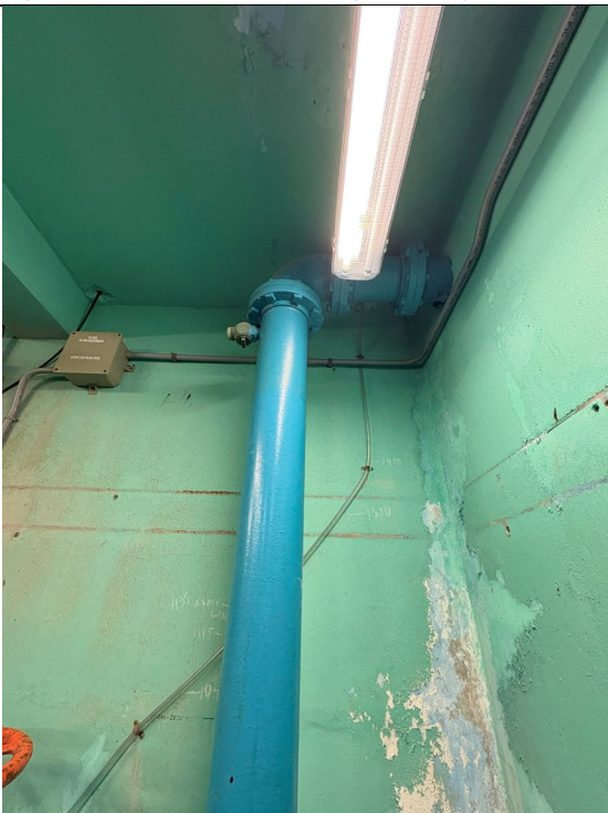
Figure 565: Gate Valve and Check Valve
