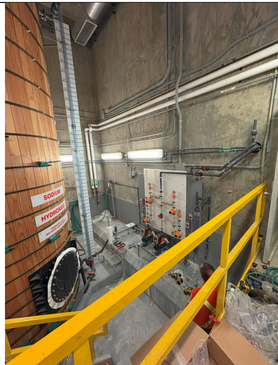
Figure 16: Sodium Hydroxide Pumps, Piping & Controls
