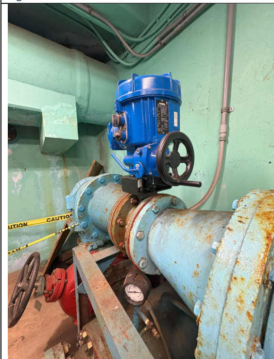
Figure 569: Butterfly Valve and Feed to Booster Pumps
