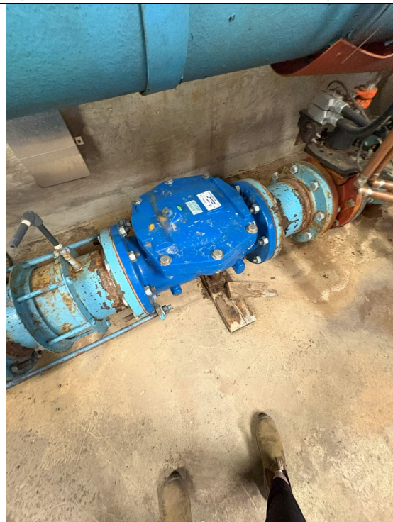
Figure 166: Check Valve
