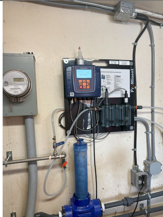
Figure 498: Chlorine Monitor
