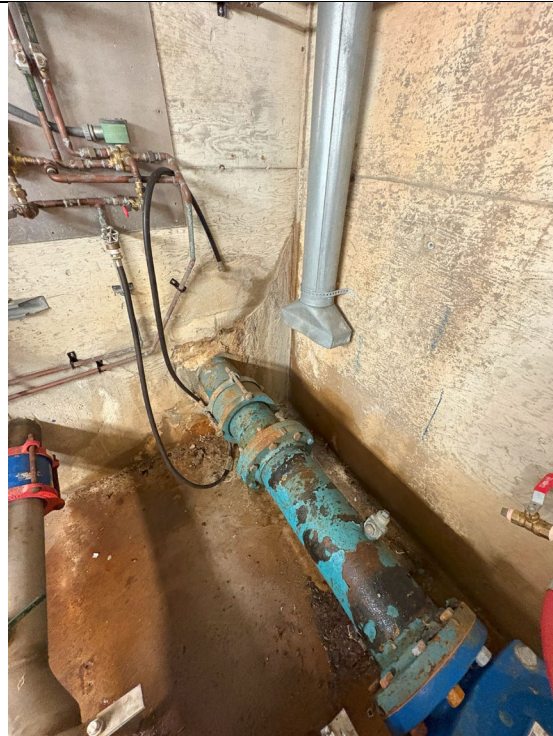
Figure 303: Corrosion of Pipe
