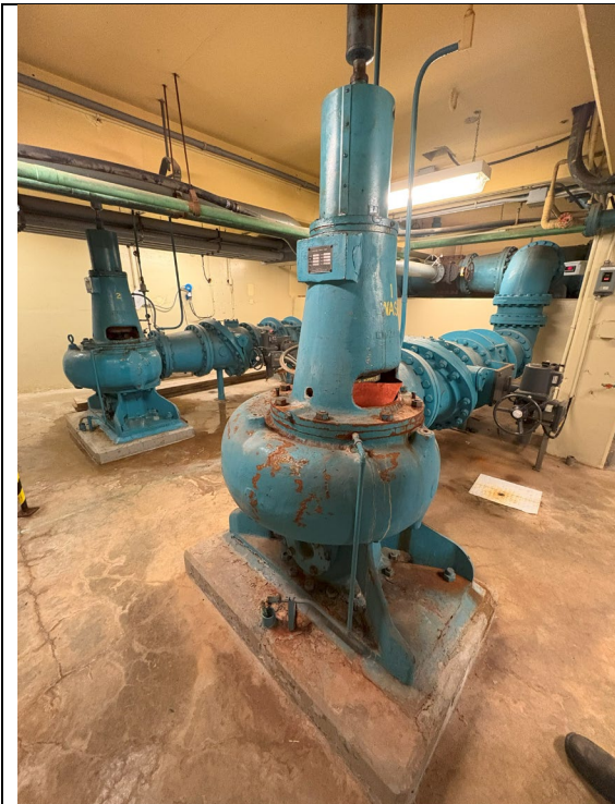
Figure 77: High Lift Pump #1 & #2
