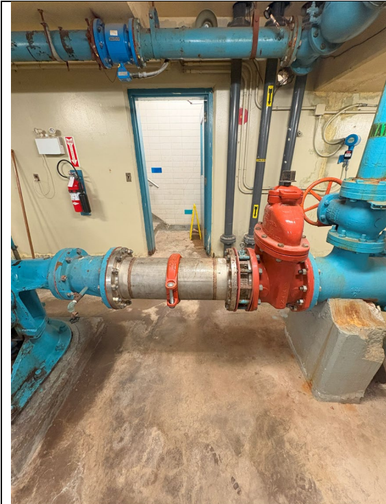
Figure 69: Gate Valve High Lift Pump #1
