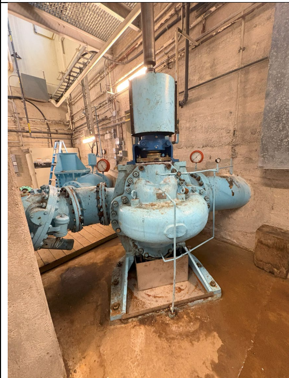
Figure 7: Electric Low Lift Pump #3
