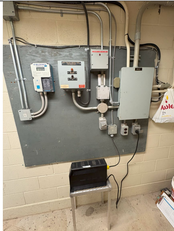
Figure 531: Control Panel in Valve Room
