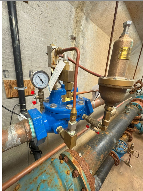
Figure 323: 2" Pressure Reducing Valve
