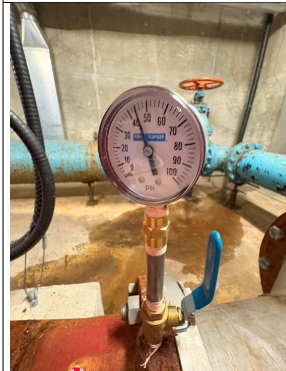
Figure 161: Inlet Pressure Pump #2
