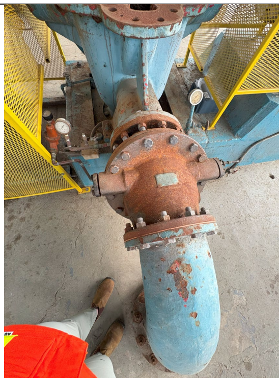
Figure 402: Pump #4 Check Valve
