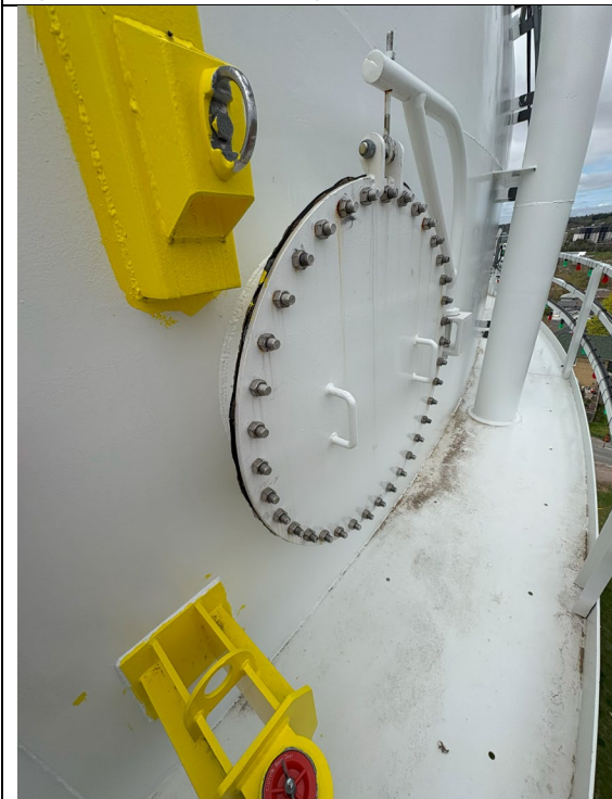
Figure 459: Water Tower Hatch
