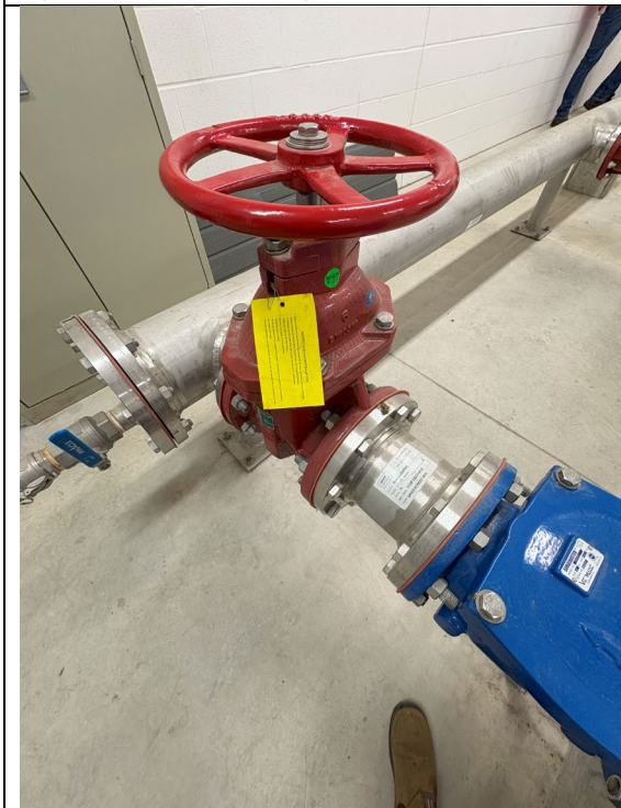
Figure 284: Discharge Gate Valve Pump #2
