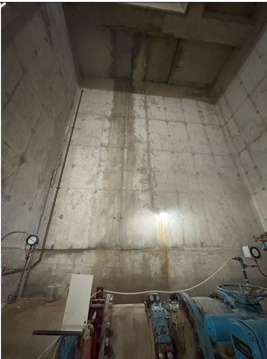
Figure 621: Pipe Room Ceiling, Surface Water Leaking
