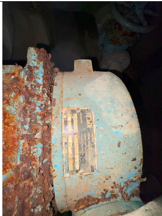
Figure 606: Corrosion Occurring on Process Piping
