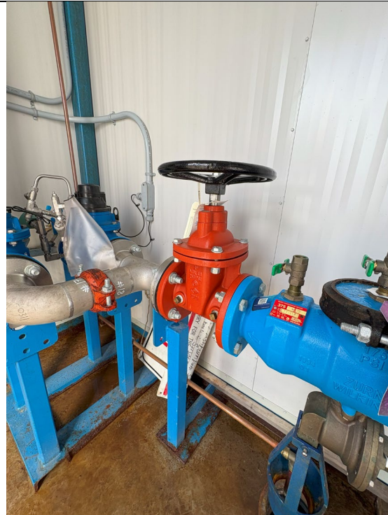
Figure 636: Gate Valve on Backflow Preventer
