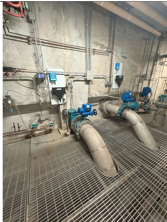
Figure 46: Filter Bed #3 Piping
