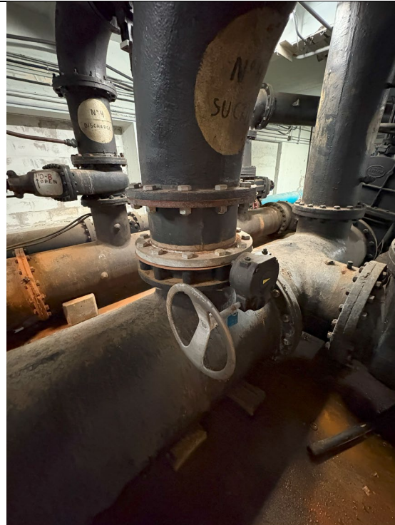
Figure 374: Pump 4 Suction Butterfly Valve
