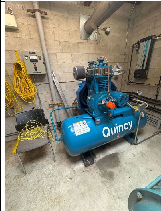
Figure 91: Air Compressor
