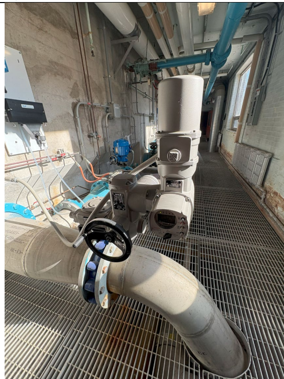
Figure 54: Drain Actuator Installed on Filter #9
