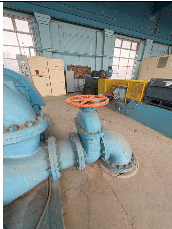
Figure 396: Pump #5 12" Gate Valve
