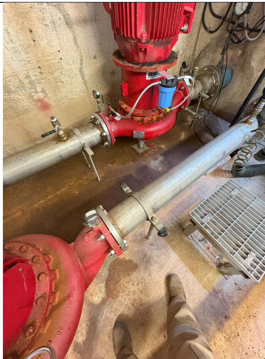
Figure 301: Discharge Pipe Pump #2
