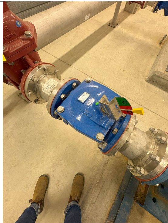
Figure 283: Check Valve at Discharge of Pump #2
