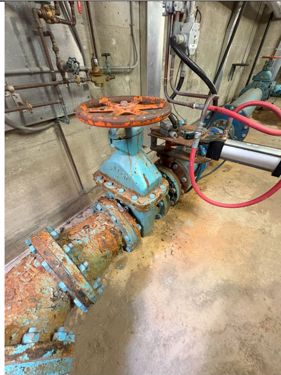
Figure 156: Butterfly Valve on Pump #1
