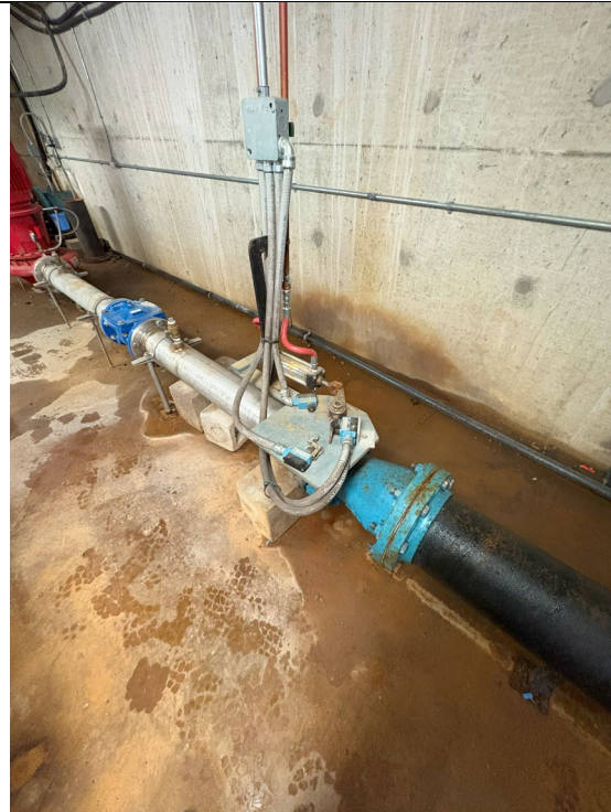
Figure 184: Check Valve & Reducer
