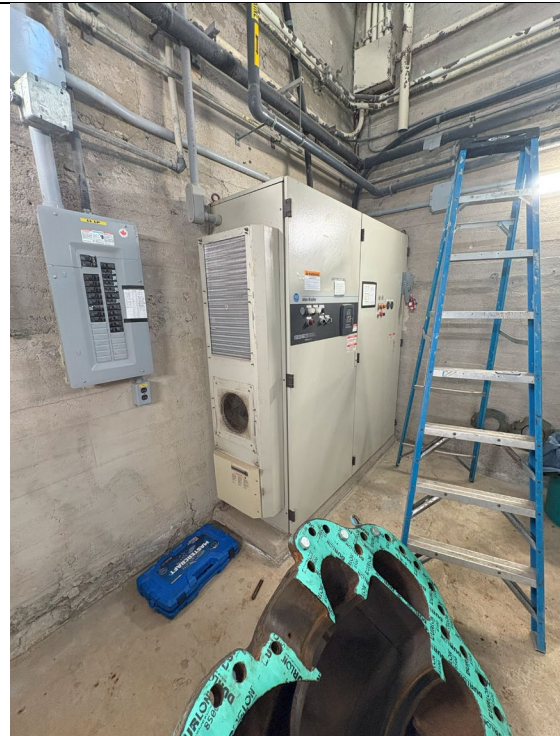
Figure 12: Low Lift Pump MC
