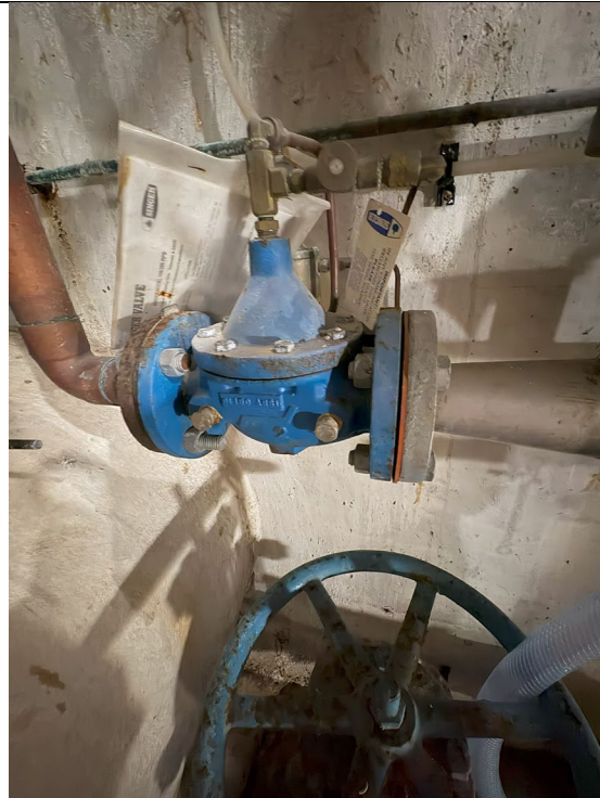
Figure 624: Pressure Relief Valve
