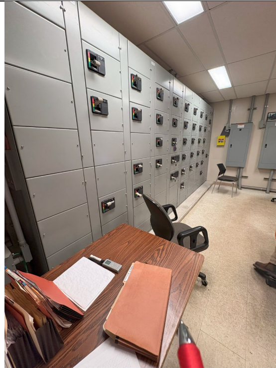
Figure 142: Electrical Switch Gear
