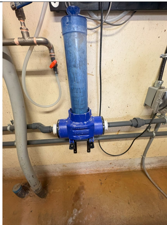
Figure 506: Valve Room Chlorinator
