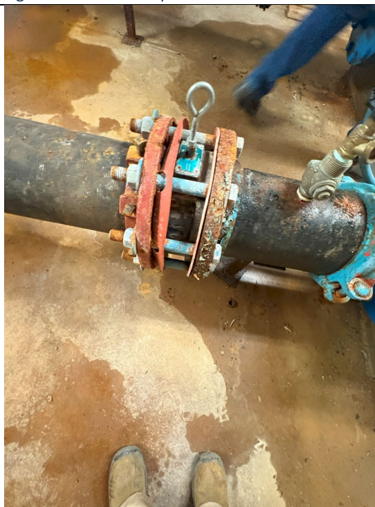
Figure 194: Coupling
