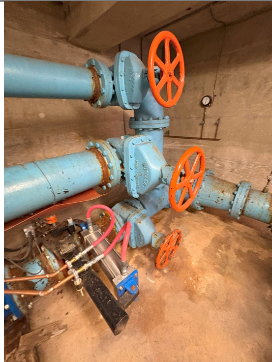
Figure 168: Gate Valves
