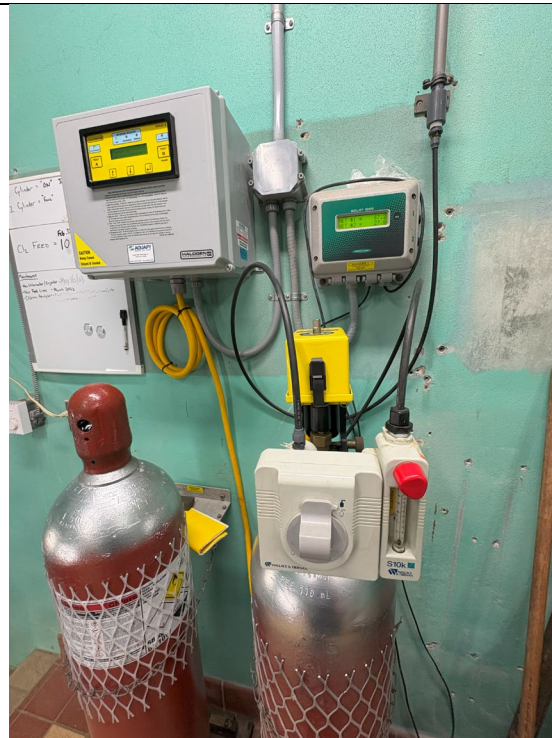
Figure 592: Chlorine Injection System
