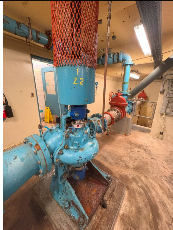
Figure 70: High Lift Pump #1
