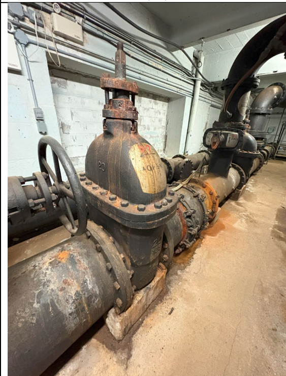
Figure 364: Gate Valve (D7)
