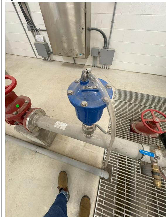
Figure 288: Air Release Valve
