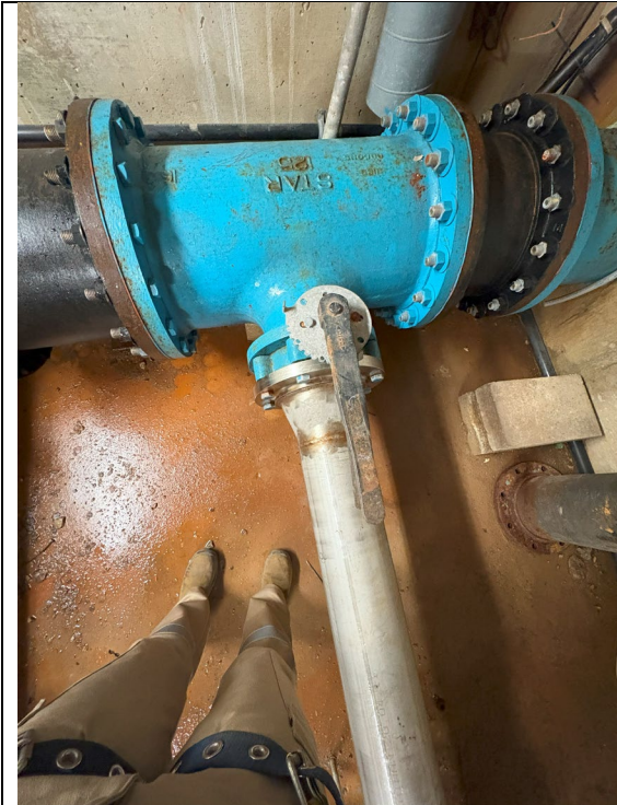
Figure 187: Butterfly Valve on Pump #1
