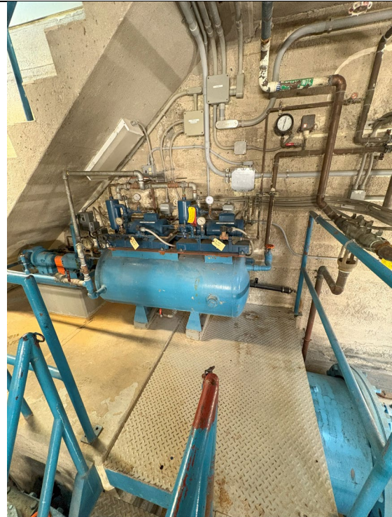
Figure 10: Vacuum Pumps
