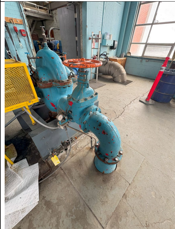
Figure 423: 8" Gate Valve on Pump #1
