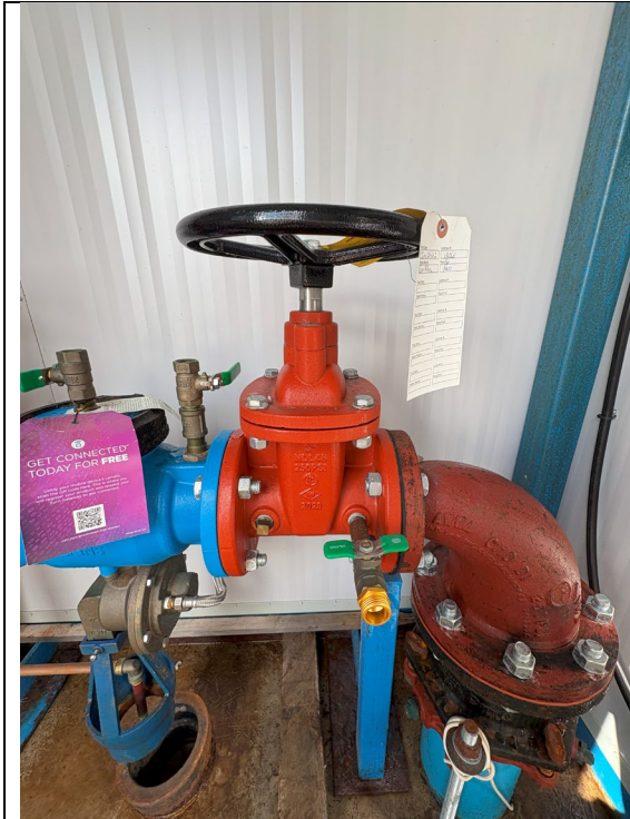
Figure 635: Gate Valve on Backflow Preventer
