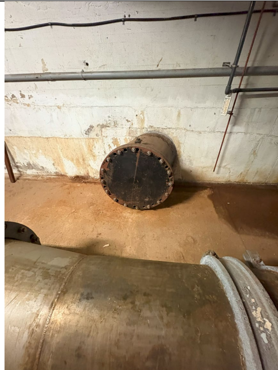
Figure 355: North Wall Historical Emergency Inlet Capped
