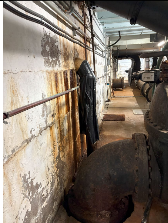
Figure 343: North Wall Water Damage
