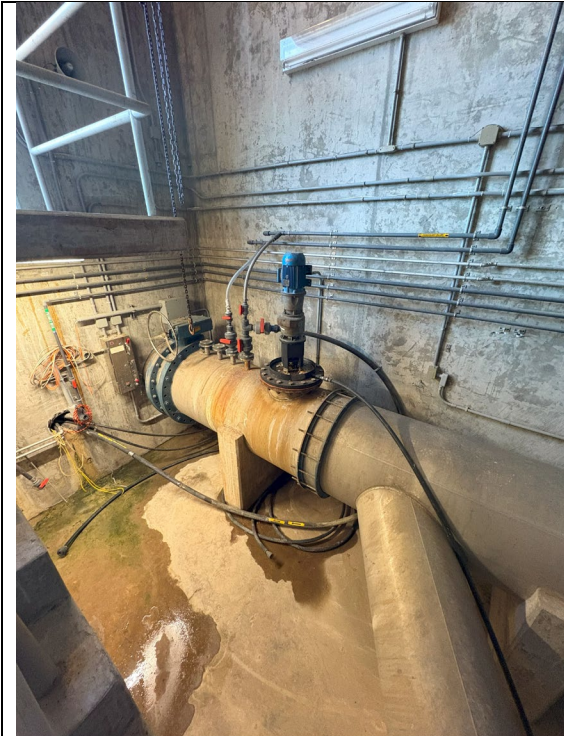
Figure 13: Raw Water Piping, Coagulation Injection Point
