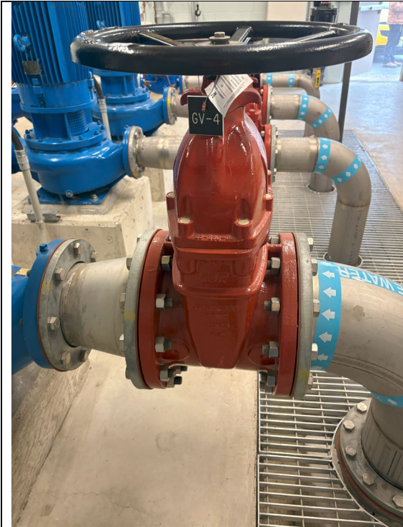
Figure 239: Gate Valve #4
