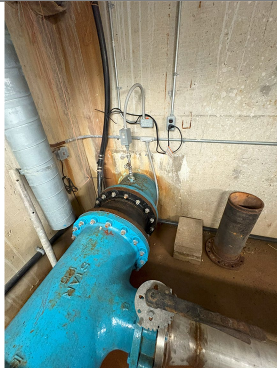
Figure 188: Piping Tee
