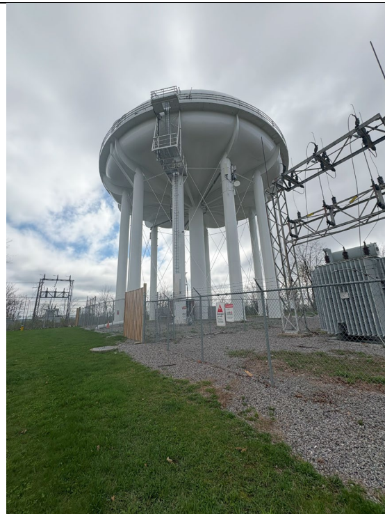
Figure 434: Elevated Tank Exterior Coating
