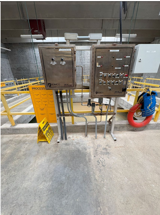
Figure 23: Sedimentation Basin 5 & 6 Controls
