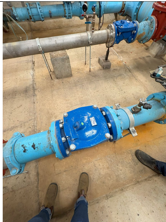
Figure 249: Check Valve on Pump #1
