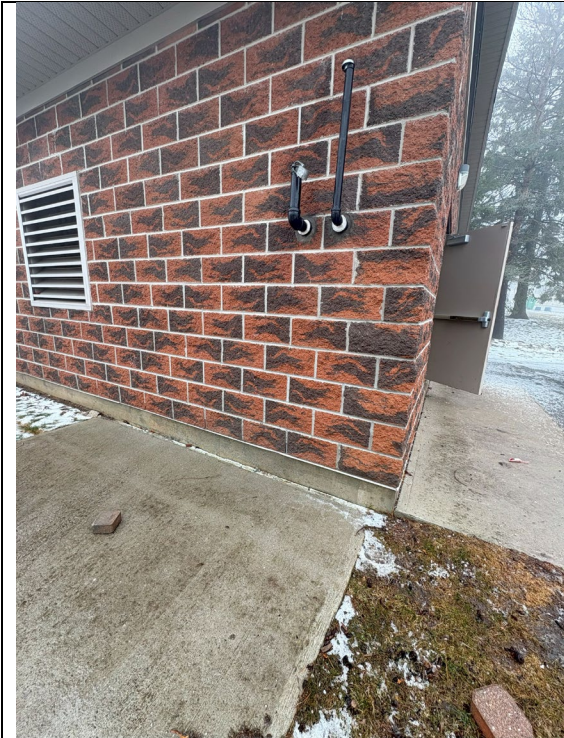
Figure 211: Generator Fueling Station
