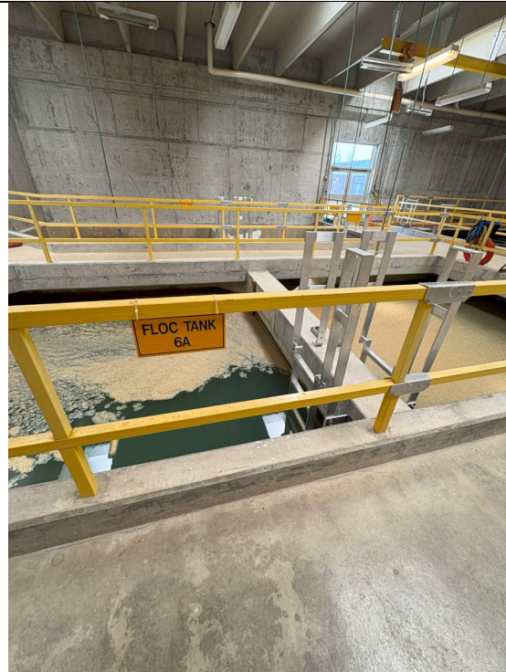
Figure 26: Flocculation Tank 6A
