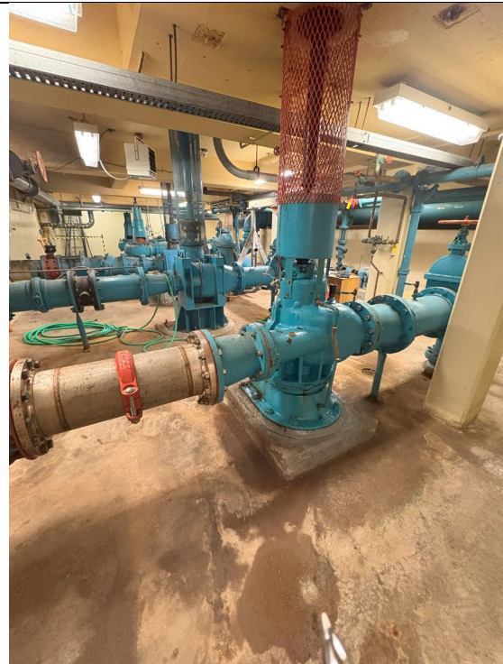
Figure 71: High Lift Pumps at Water Treatment Plant
