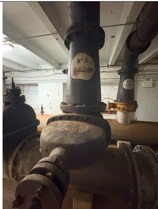
Figure 349: Pump #2 Suction Gate Valve
