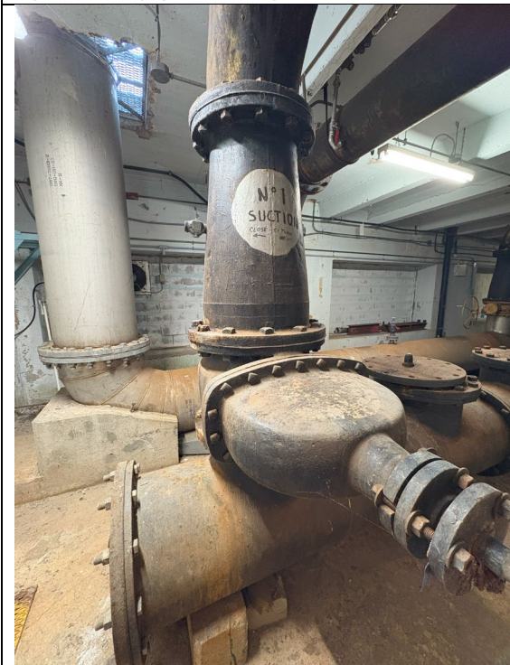
Figure 344: Pump #1 Suction Gate Valve
