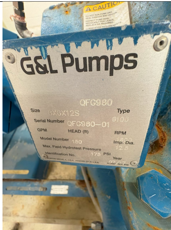
Figure 277: Label on Pump #1
