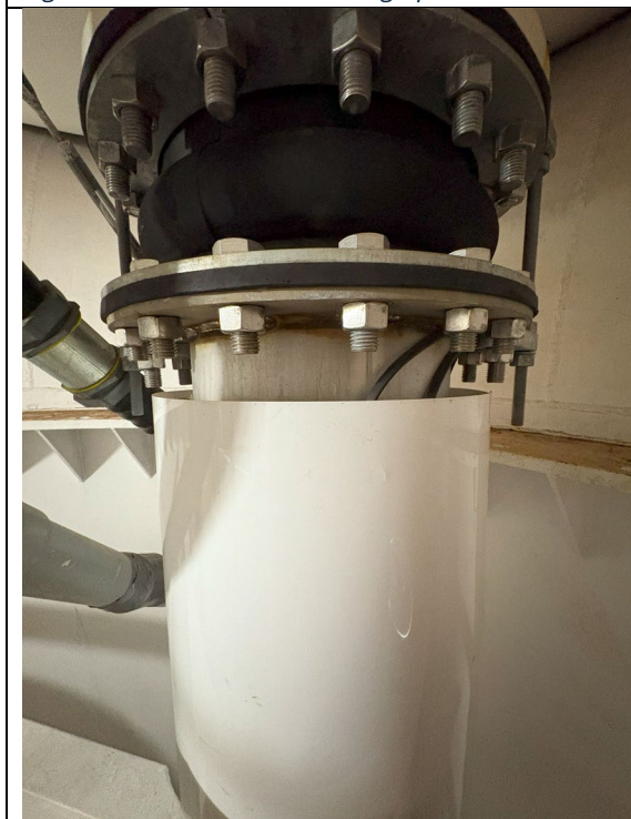
Figure 479: Process Piping Insulation
