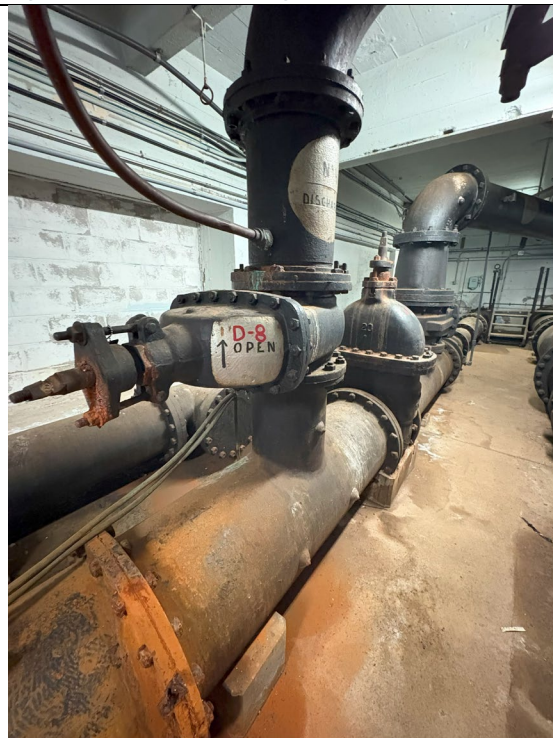
Figure 365: Gate Valve (D8)
