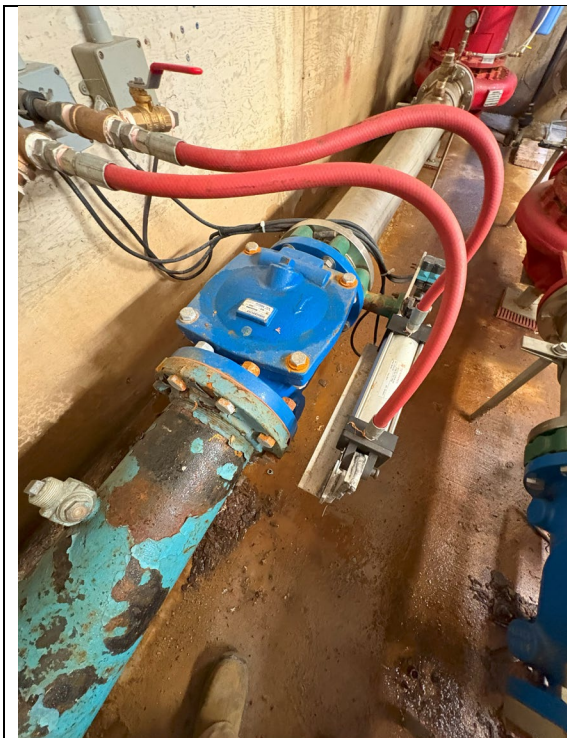
Figure 306: Butterfly Valve and Check Valve Pump #1
