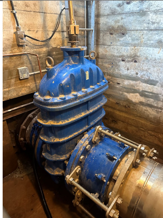
Figure 446: 500mm Gate Valve
