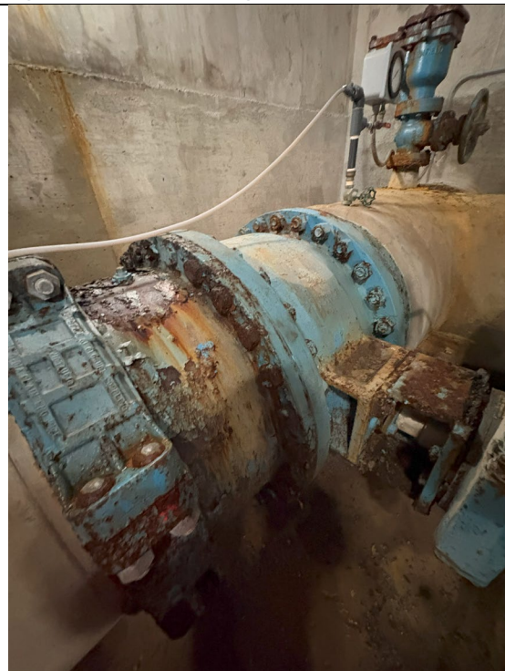
Figure 610: Corrosion Occurring on Process Piping
