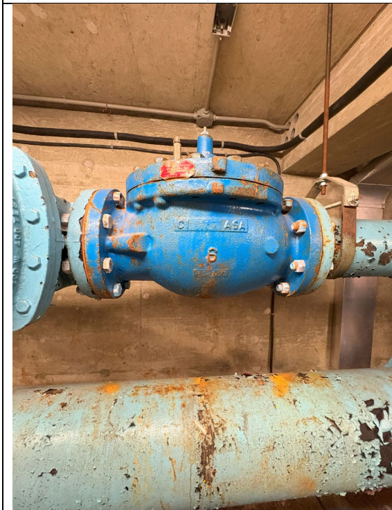
Figure 165: Pressure Reducing Valve
