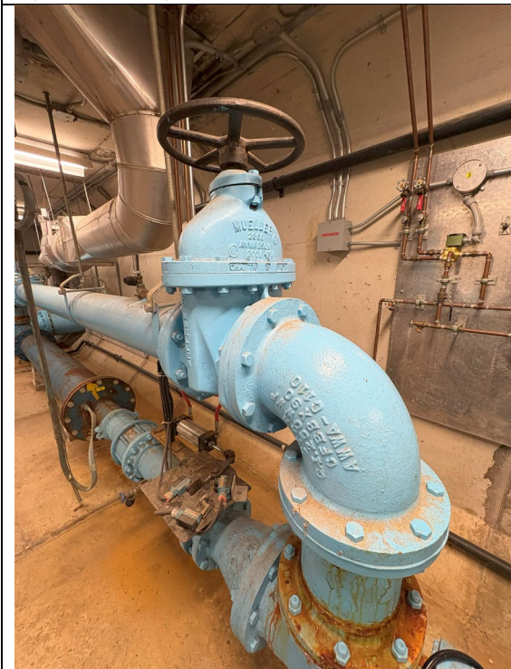
Figure 264: Discharge Gate Valve on Pressure Relief
