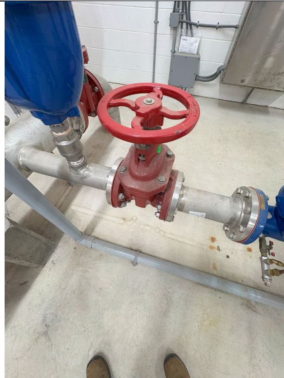
Figure 291: Suction Gate Valve on PRV
