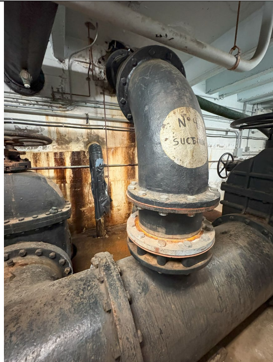
Figure 369: Pump #4 Suction
