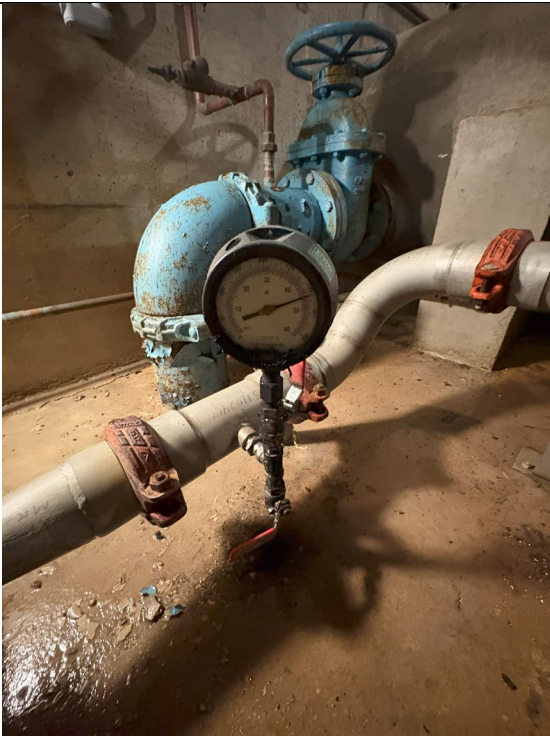
Figure 613: Pressure Gauge
