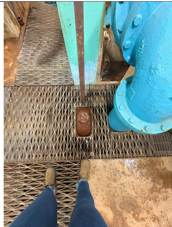
Figure 581: 12" Gate Valve
