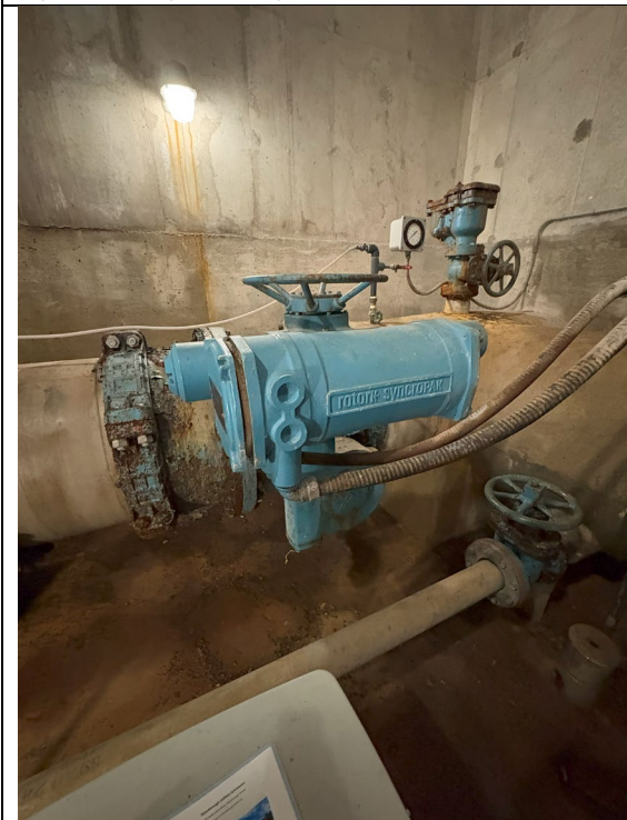
Figure 605: Actuator for Valve
