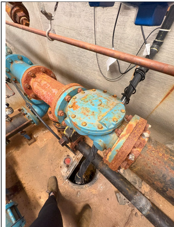
Figure 324: Check Valve on By-Pass
