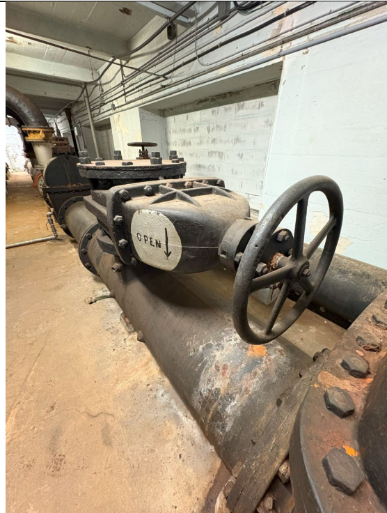
Figure 366: Pump #4 Discharge Gate Valve (D8)
