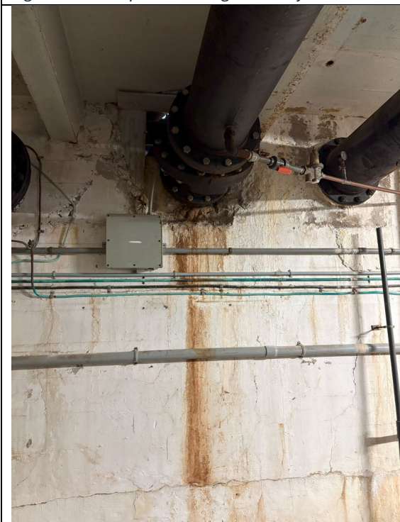
Figure 352: Pump #2 Discharge Check Valve
