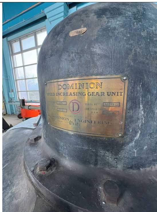
Figure 426: Label on Pump #1 Gear Increaser
