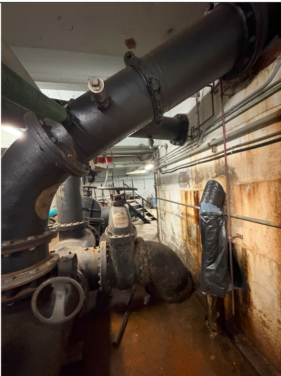
Figure 375: Pump #4 Suction Pipe
