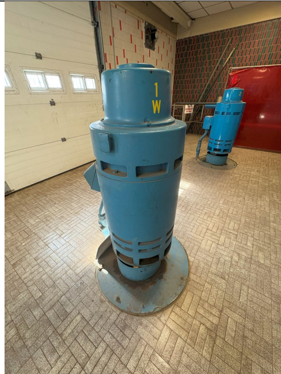
Figure 66: Backwash Electric Motor #1
