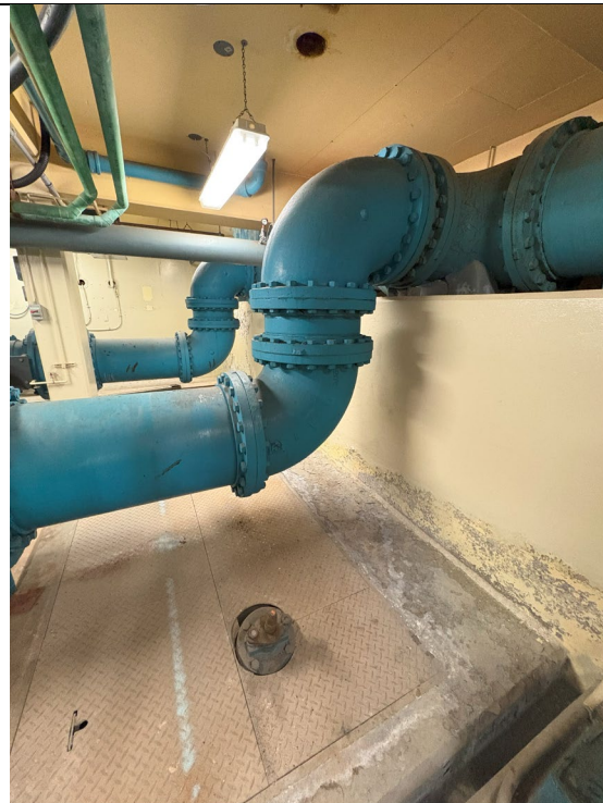
Figure 78: High Lift Pump Piping
