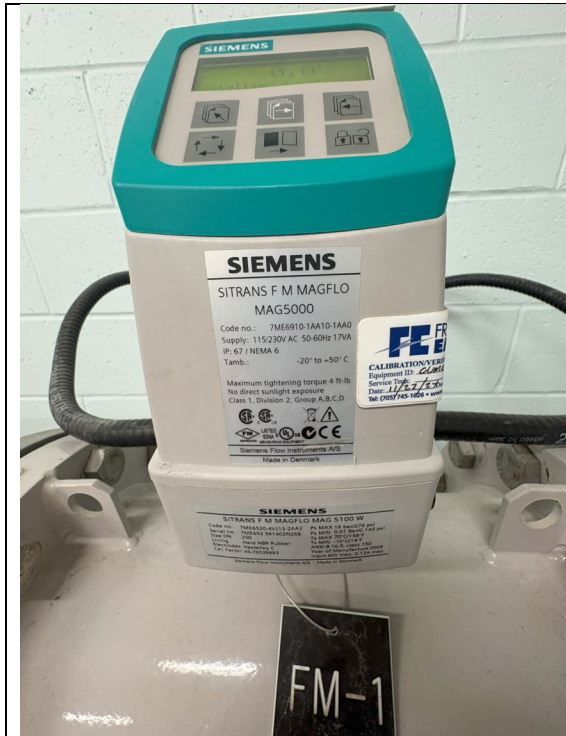
Figure 223: Siemens Flow Meter
