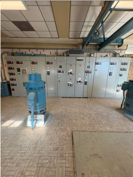
Figure 67: Electrical Panel and MCC
