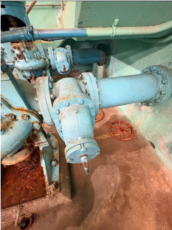
Figure 577: Check Valve Pump #2
