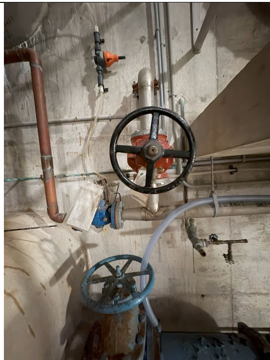
Figure 618: Gate Valve
