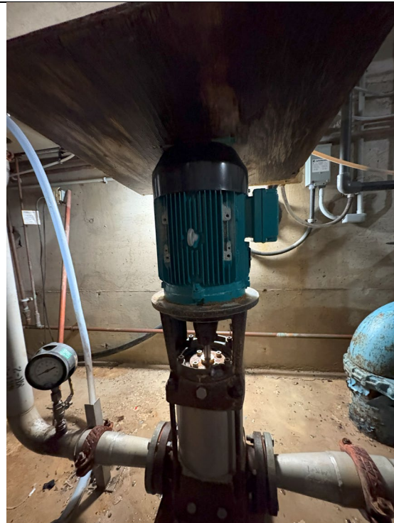
Figure 614: Pump for Flushing the Reservoir
