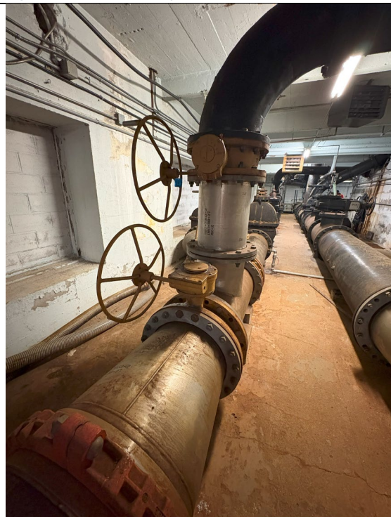
Figure 356: Butterfly Valves
