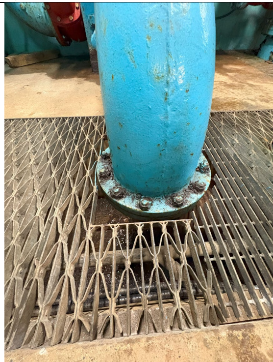
Figure 582: Corrosion on Flange
