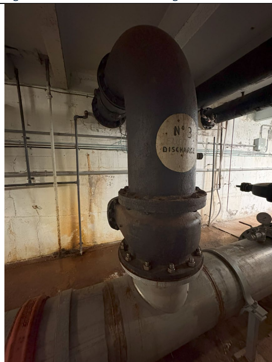
Figure 353: Pump#3 Suction Gate Valve (labelled incorrectly)
