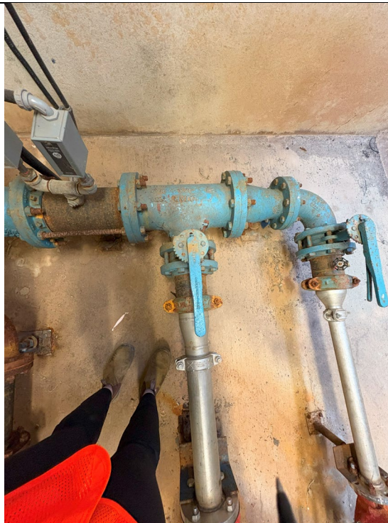
Figure 329: Butterfly Valves on Pump 1 & 2
