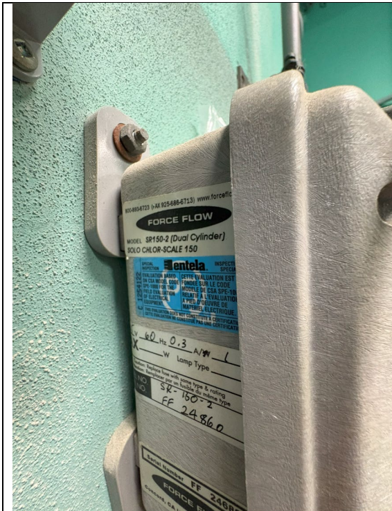
Figure 591: Label on Chlorine Scale
