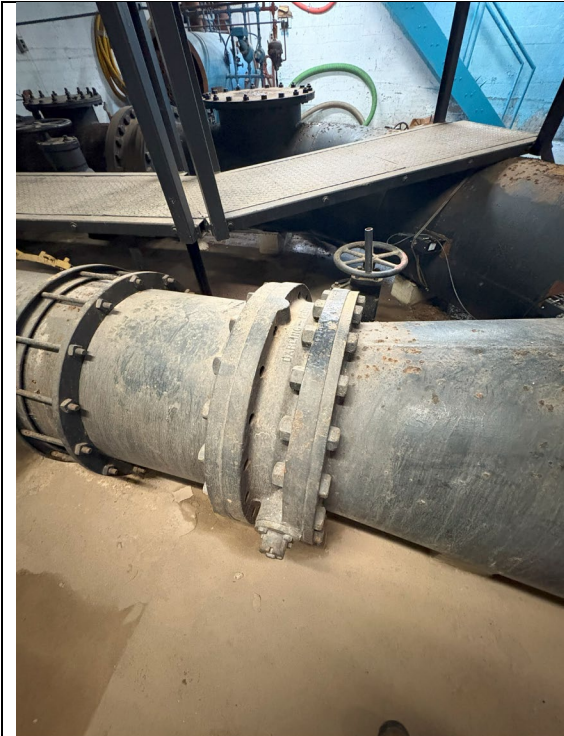
Figure 377: 24" Butterfly Valve
