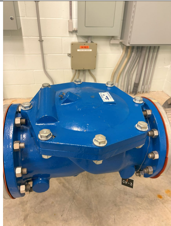
Figure 237: Check Valve #3
