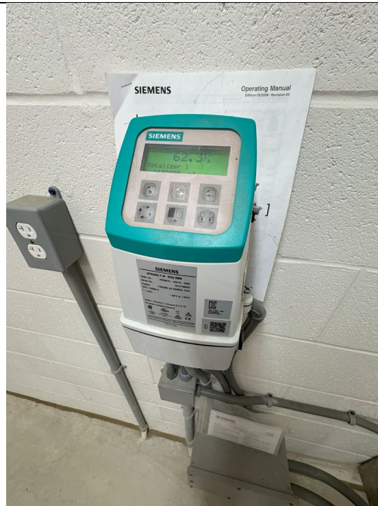
Figure 295: Siemens Flow Meter
