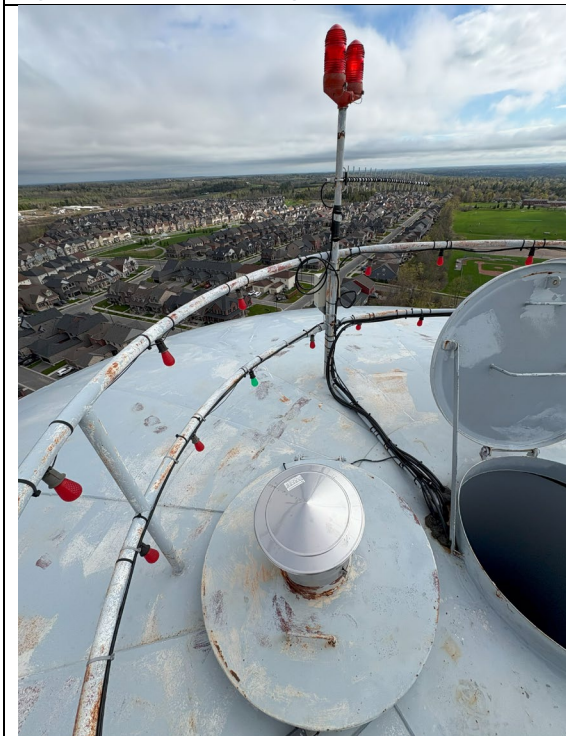
Figure 526: Breather Valve on Top of Water Tower
