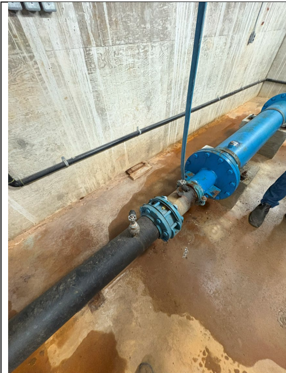
Figure 199: Coupling on Pump #3
