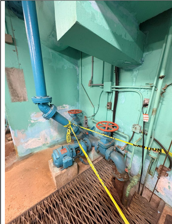
Figure 575: Pump #5 and Sump Pump
