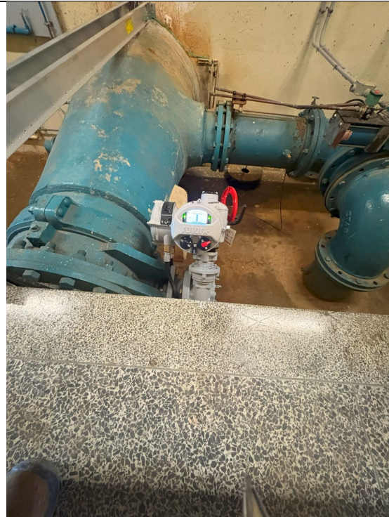
Figure 56: Filter Bed #10 Piping, New Actuator Installed
