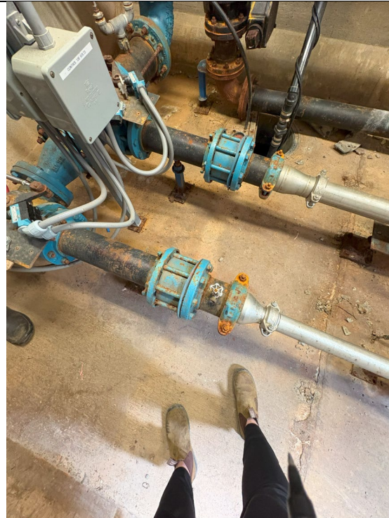
Figure 333: Reducer and Coupler Discharge from Pumps
