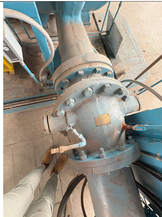
Figure 412: 10" Check Valve on Pump #3
