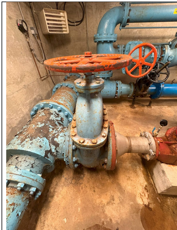
Figure 151: Gate Valve Adjacent to Pump #2
