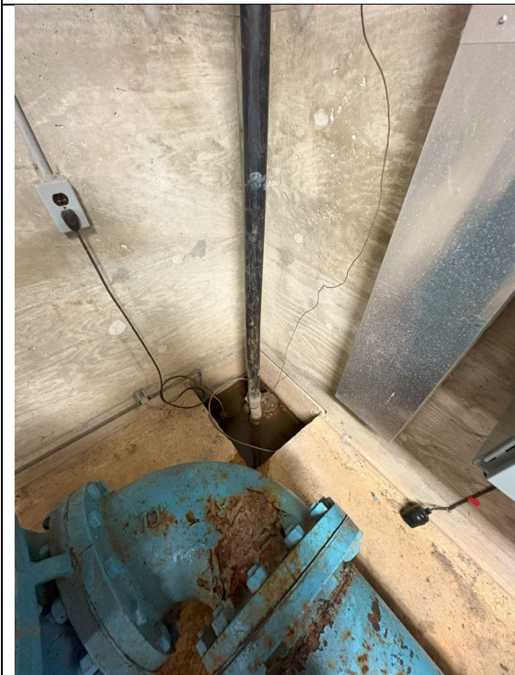
Figure 173: Sump Pit and Pump
