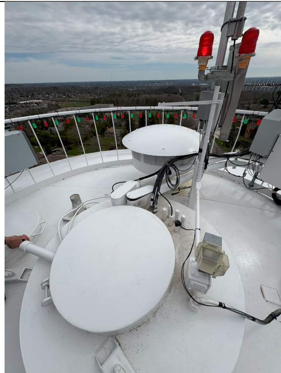
Figure 484: Ladder Access Hatch and Breather Vent
