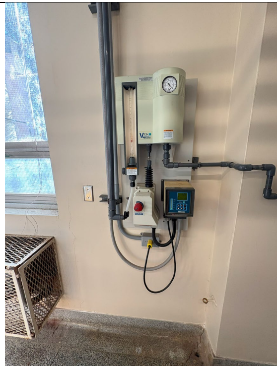
Figure 87: Halogen Valve System
