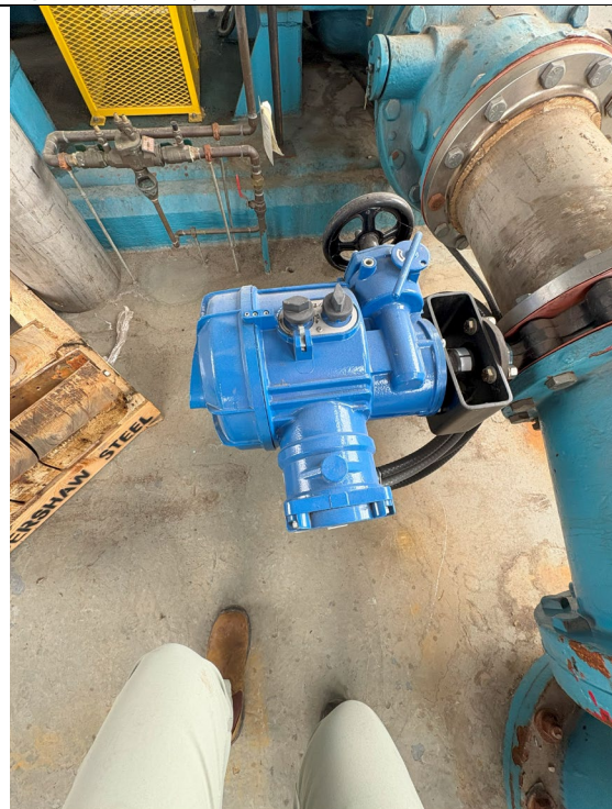
Figure 392: Butterfly Valve Upgraded Controls
