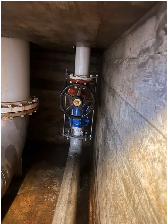
Figure 443: Gate Valve on Drainpipe
