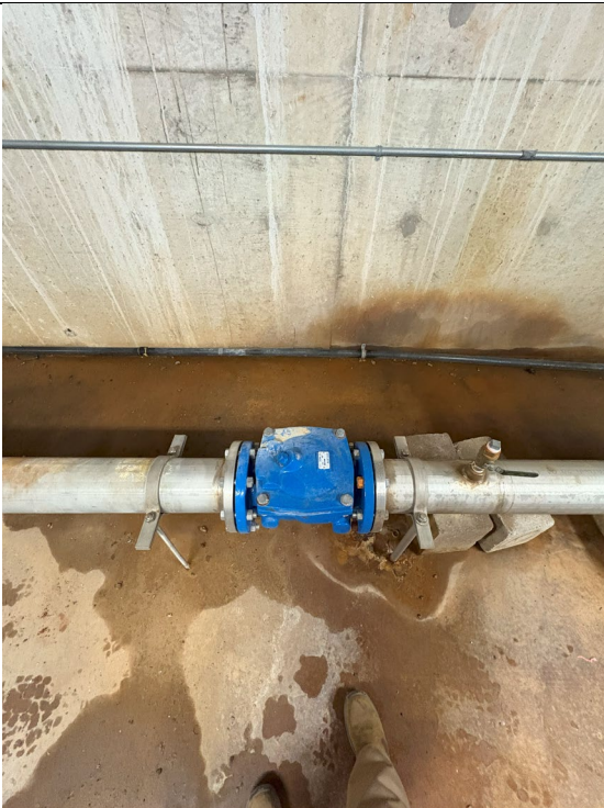
Figure 185: Check Valve
