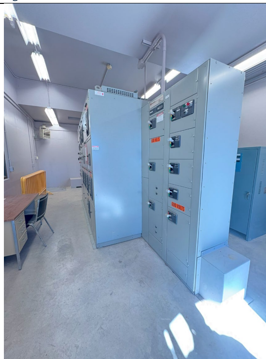
Figure 146: Electrical Switch Gear & SCADA
