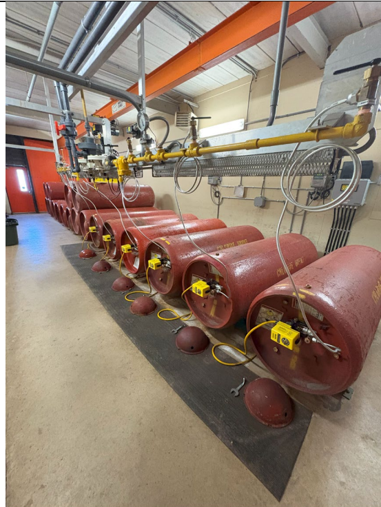
Figure 82: Chlorine Gas Cylinders
