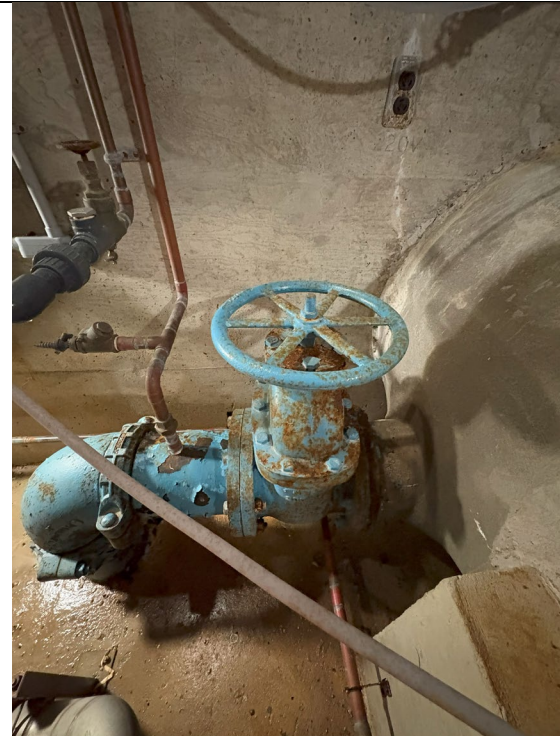
Figure 607: Gate Valve
