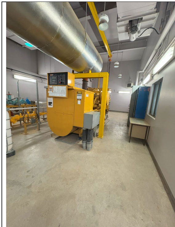
Figure 143: Caterpillar Motor with Generator Set
