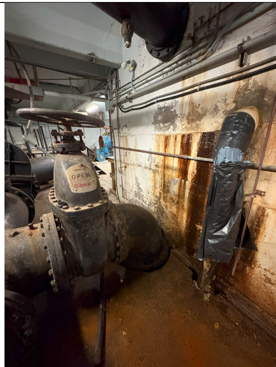
Figure 376: Darin 20" Gate Valve
