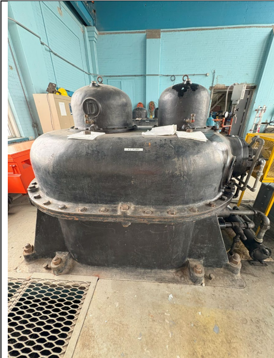
Figure 417: Gear Increaser on Pump #2
