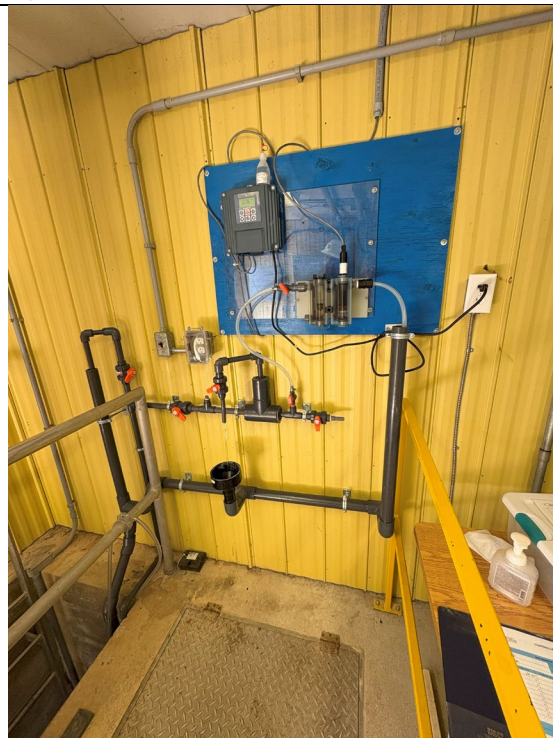
Figure 626: Chlorine Monitor
