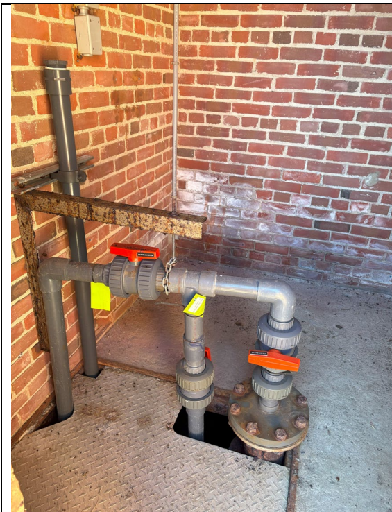
Figure 93: Chlorine Diffuser
