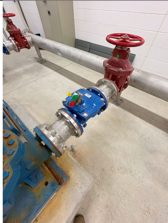
Figure 279: Check Valve & Gate Valve, Discharge of Pump #1
