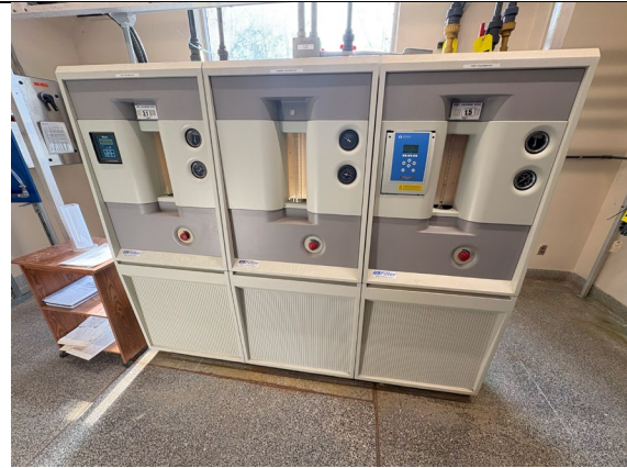
Figure 85: Primary and Secondary Disinfection Chlorination
