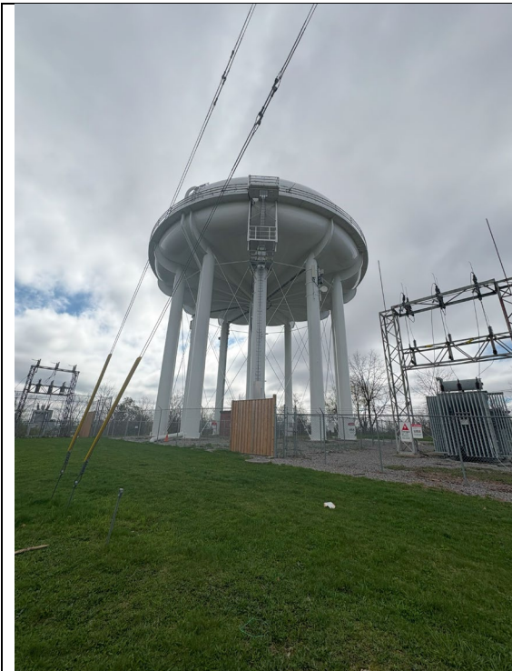
Figure 433: Elevated Tank Exterior Coating
