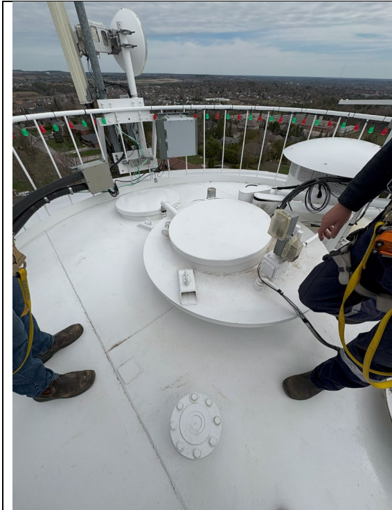
Figure 481: Hatch at Top of Tower
