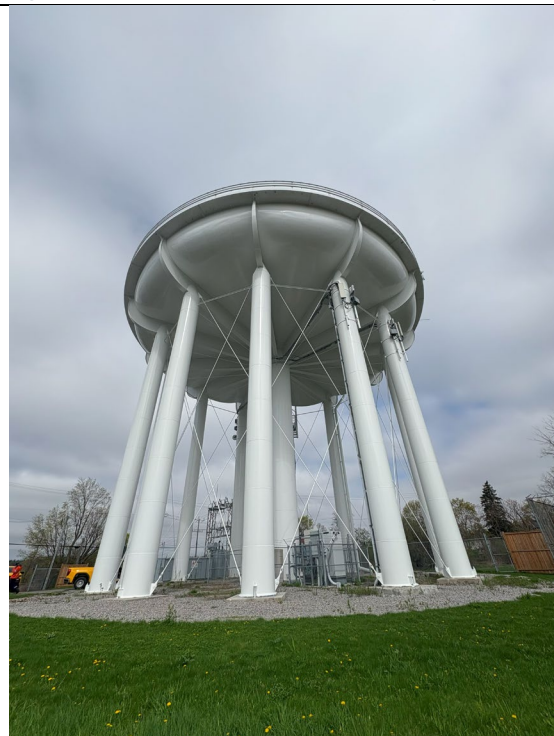
Figure 436: Elevated Tank Exterior Coating
