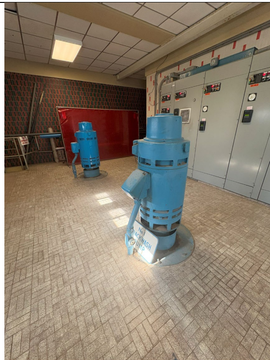
Figure 64: Backwash Electric Motor #1
