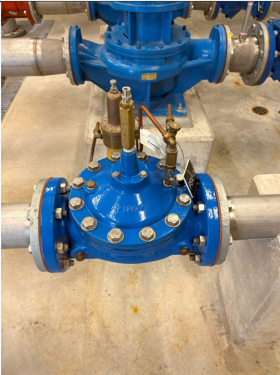
Figure 225: Pressure Relief Valve #1
