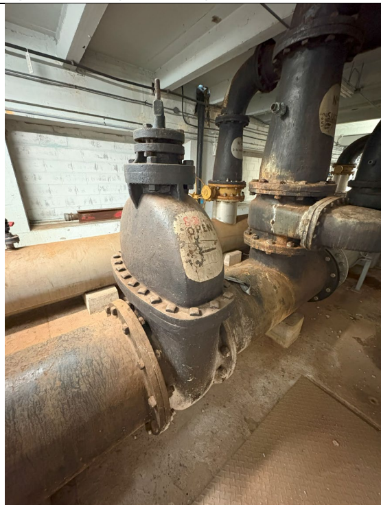
Figure 348: 20" Gate Valve
