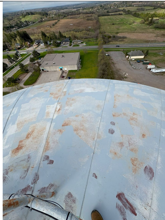
Figure 517: Exterior Coating
