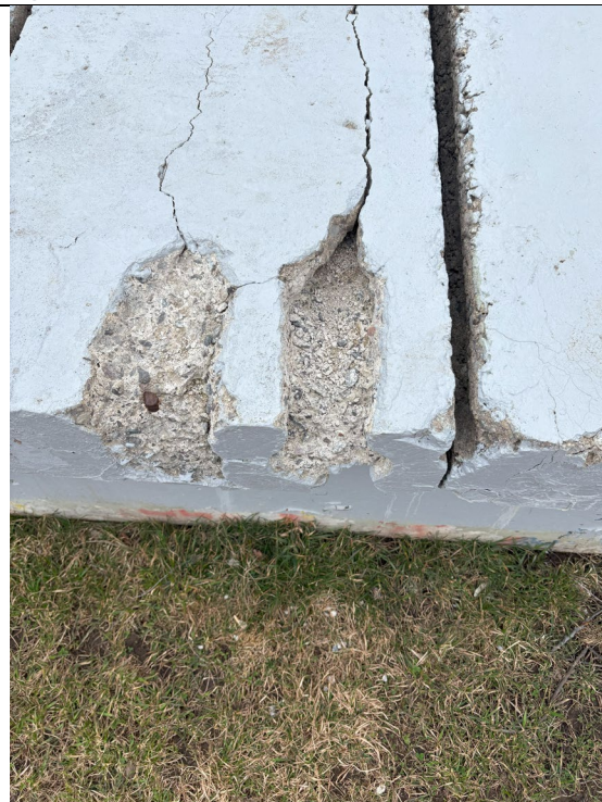
Figure 542: Deteriorated Concrete Roof
