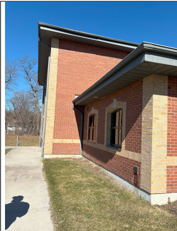
Figure 125: Exterior Eavestrough Bent
