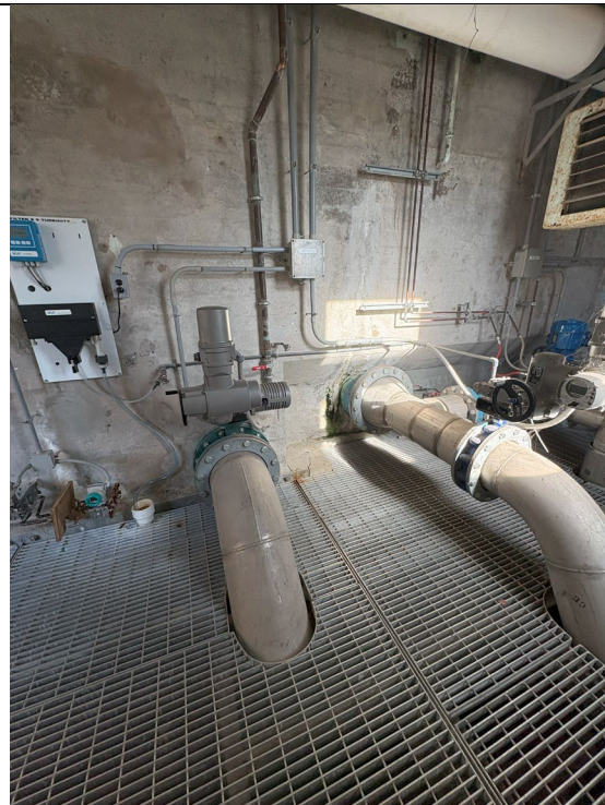
Figure 52: Filter Bed #9 Piping
