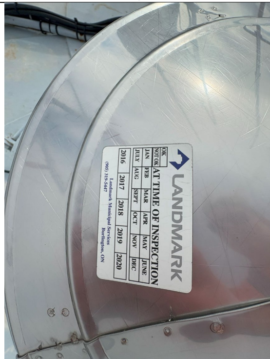
Figure 527: Breather Valve Inspection Sticker
