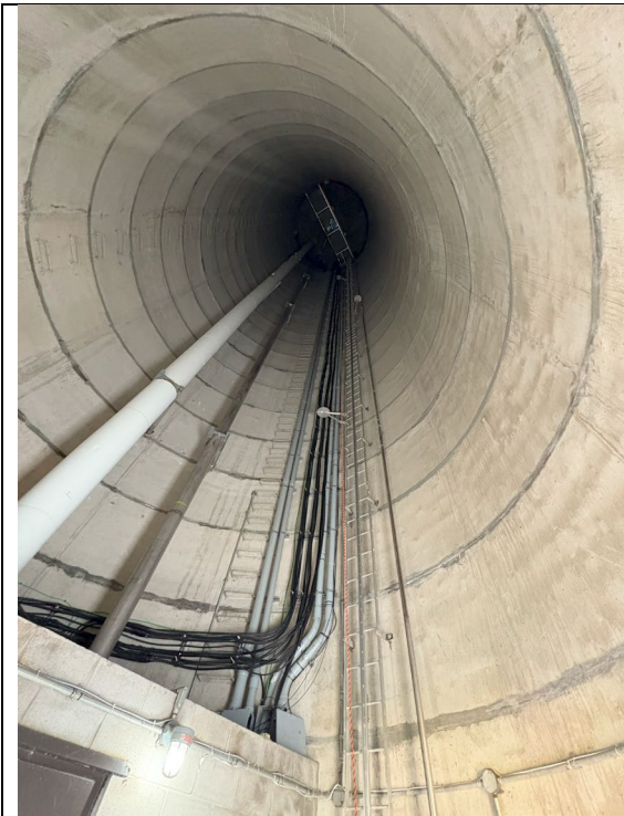
Figure 508: Looking up the Tower Inside, 12" Pipe Feed
