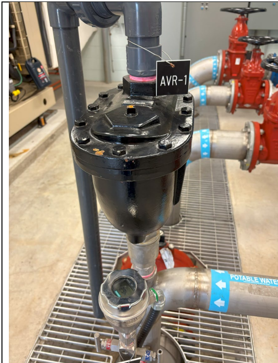
Figure 227: Air Release Valve #1
