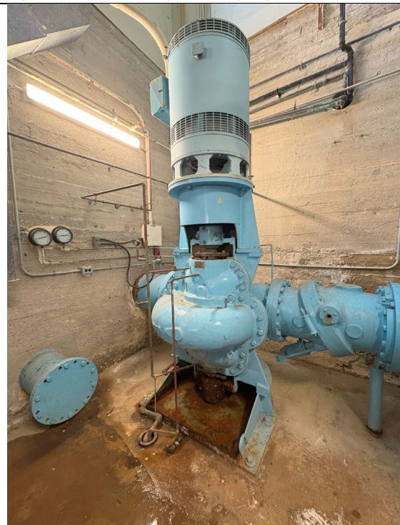
Figure 8: Electric Low Lift Pump #4
