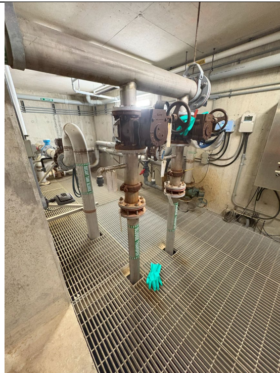
Figure 126: Sludge Tank Piping
