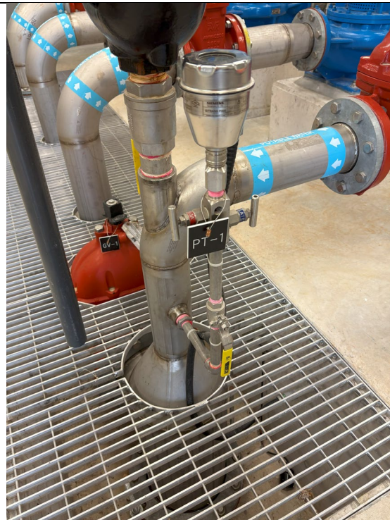
Figure 228: Pressure Gauge #1
