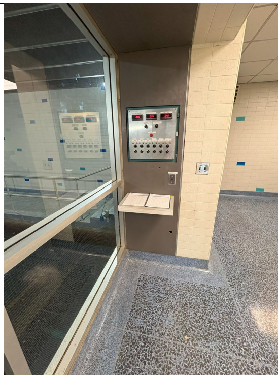
Figure 42: Filter Bed #11 Controls
