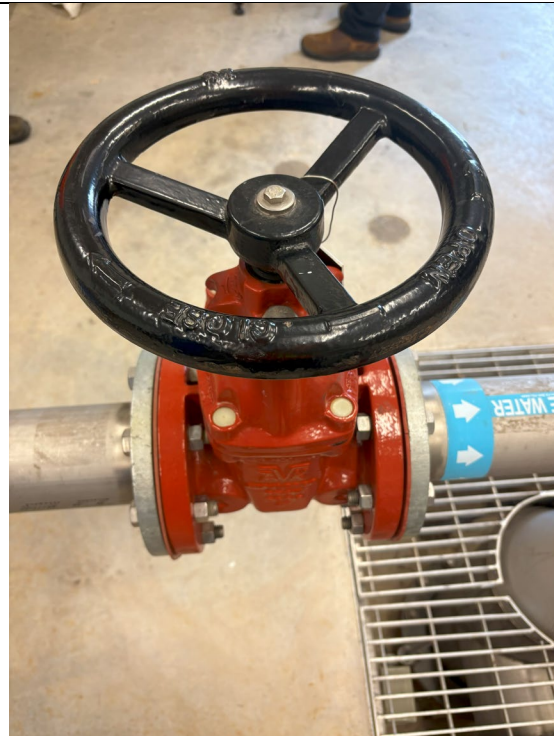
Figure 226: Gate Valve #9
