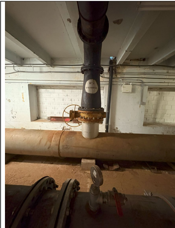
Figure 350: Pump #2 Discharge Butterfly Valve
