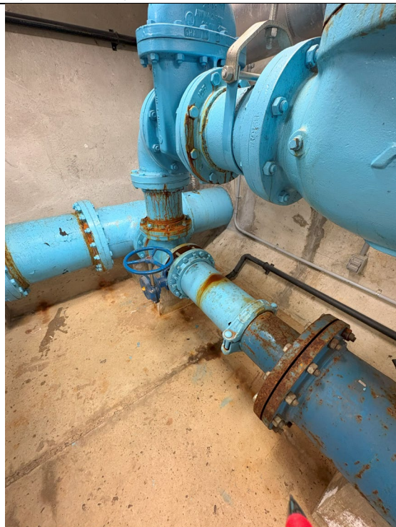
Figure 260: Corrosion on Tee
