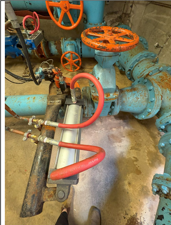
Figure 155: Butterfly Valve on Pump #2
