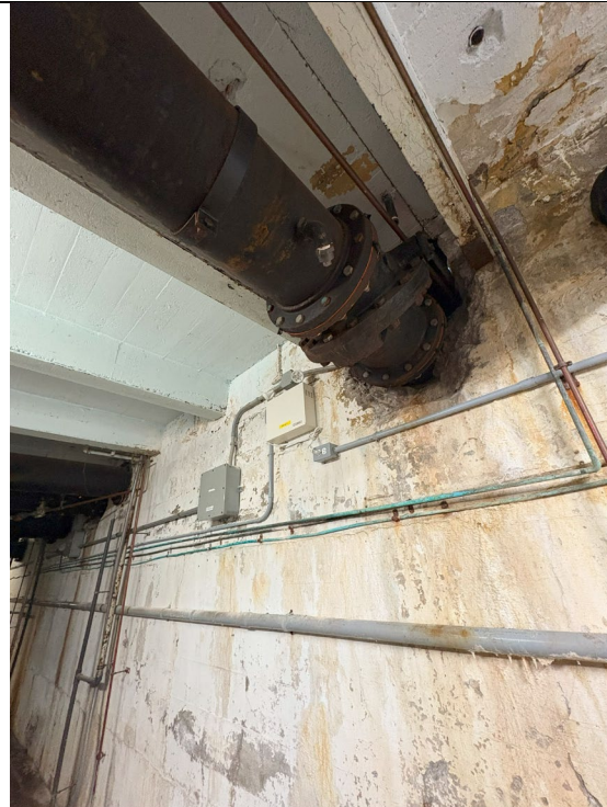
Figure 347: Pump #1 Discharge Check Valve
