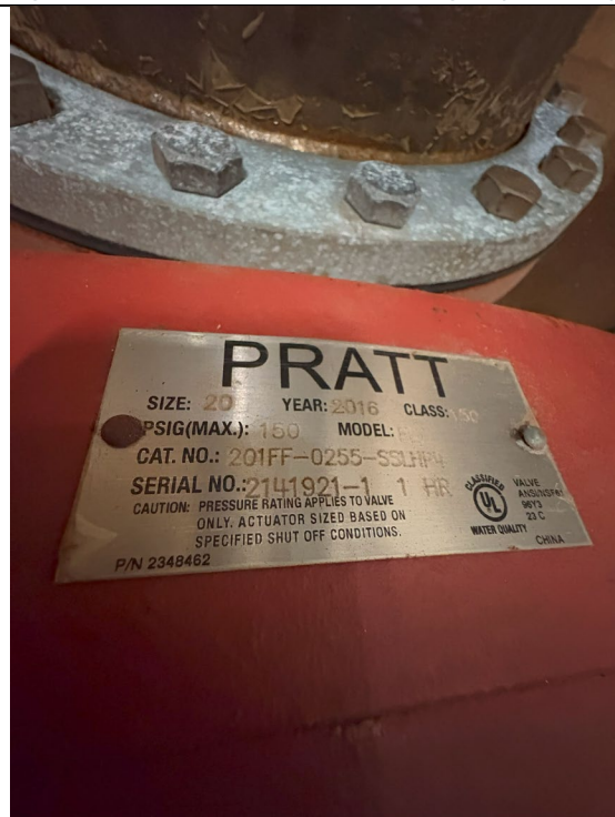
Figure 357: Label on Butterfly Valve
