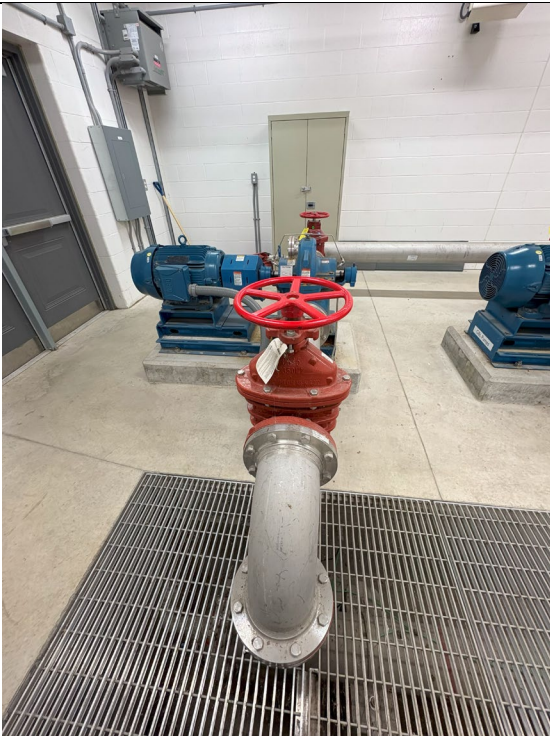
Figure 280: Suction Gate Valve on Pump #2
