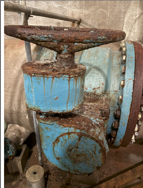
Figure 611: Corrosion Occurring on Process Piping
