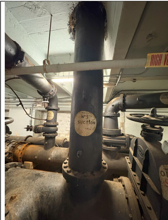
Figure 385: Pump #5 Suction Pipe
