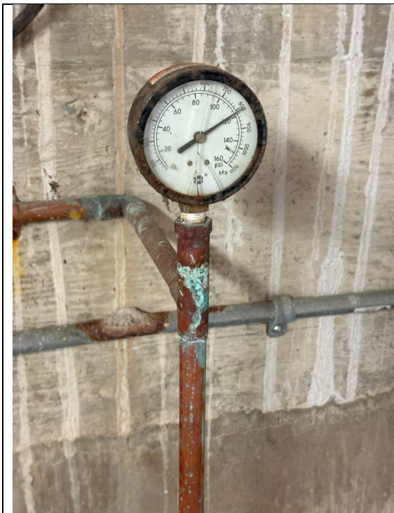
Figure 179: Discharge Pressure Gauge
