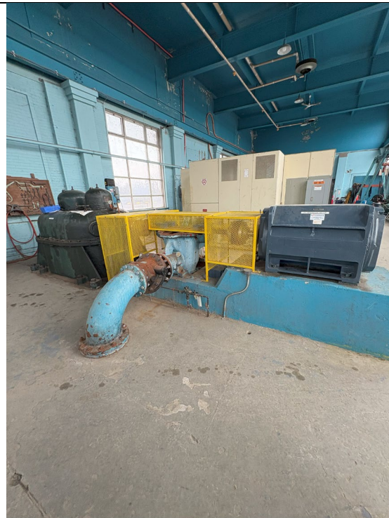
Figure 398: Pump #4 & Generator (can be setup as a motor)
