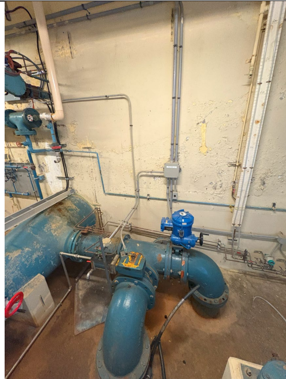
Figure 60: Filter Bed #11 Piping, New Actuator Installed
