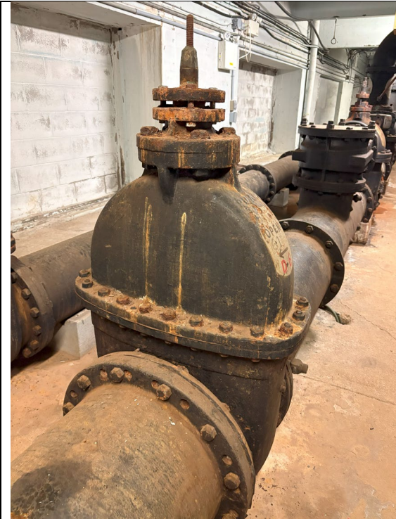
Figure 362: 20" Gate Valve (D6)
