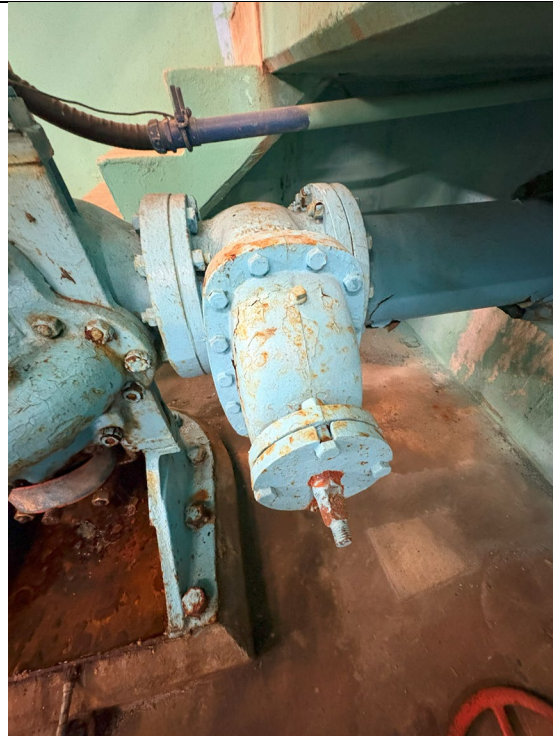
Figure 576: Check Valve Pump #1
