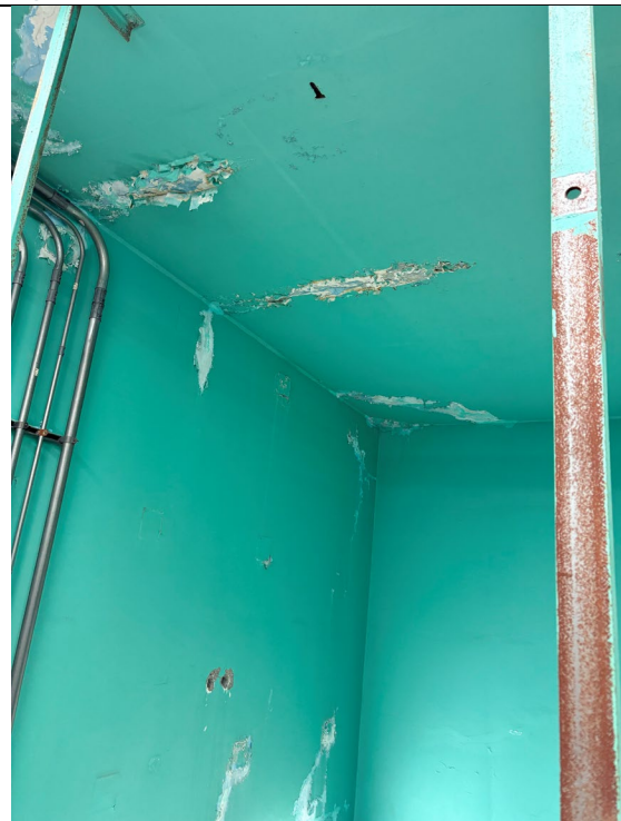
Figure 593: Peeling Paint
