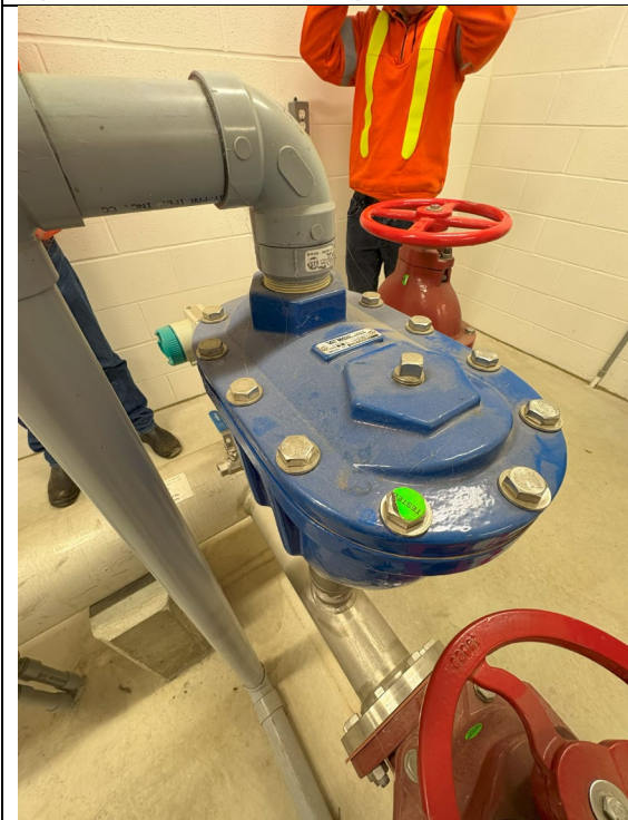
Figure 292: Air Release Valve
