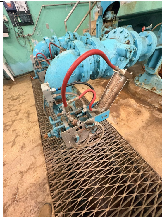
Figure 554: Hydraulic Butterfly Valve on Pump #2
