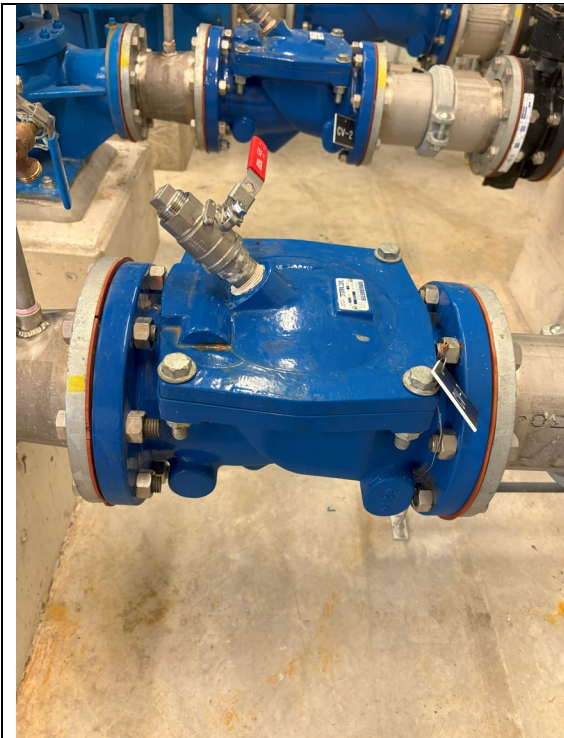
Figure 231: Check Valve #1
