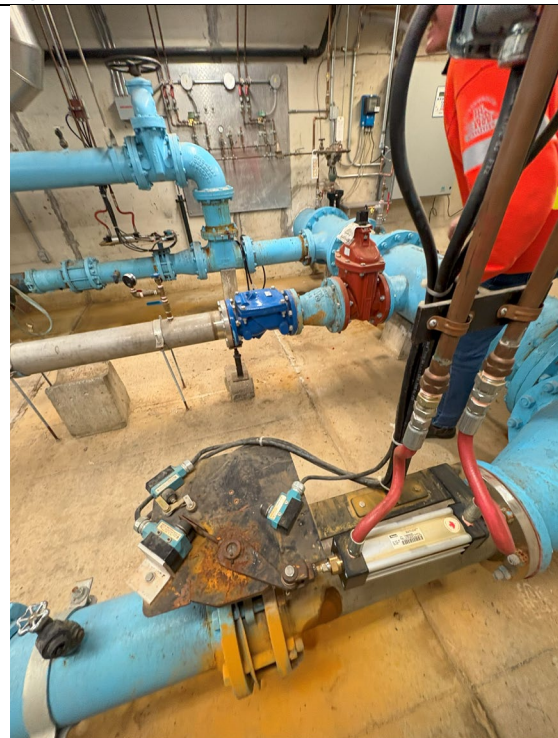
Figure 248: Butterfly Valve on Pump #1
