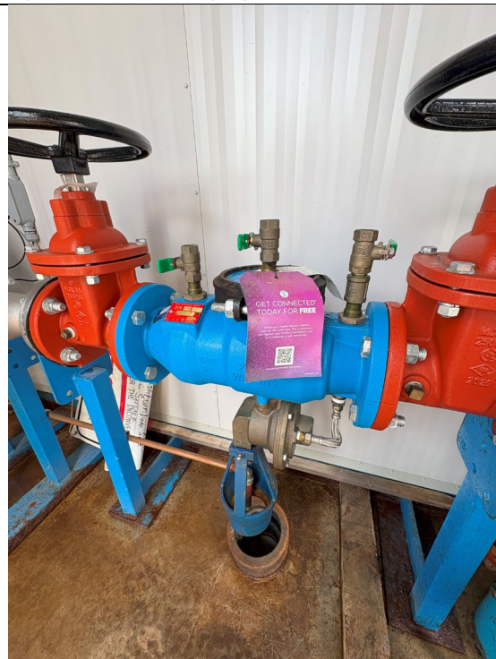
Figure 634: Backflow Preventer
