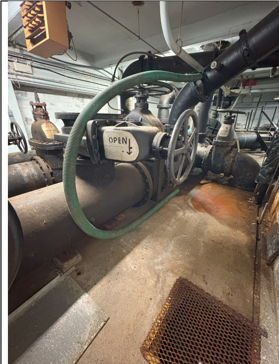
Figure 373: Out of Use Gate Valve
