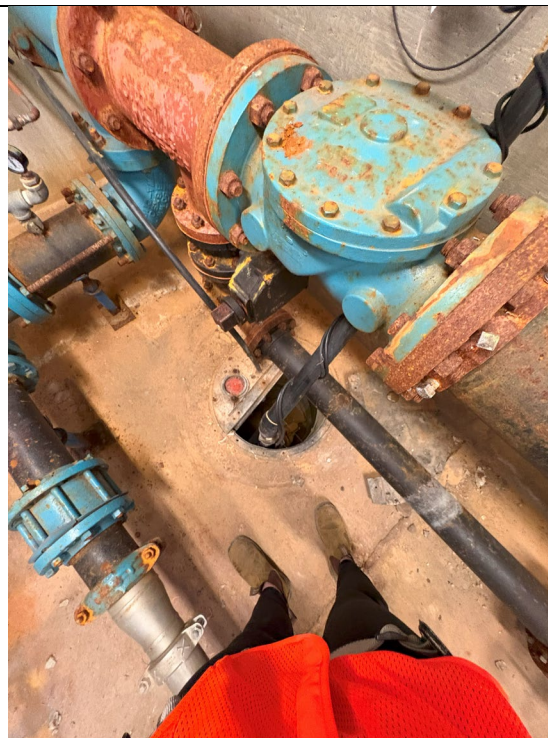
Figure 325: Sump Pump
