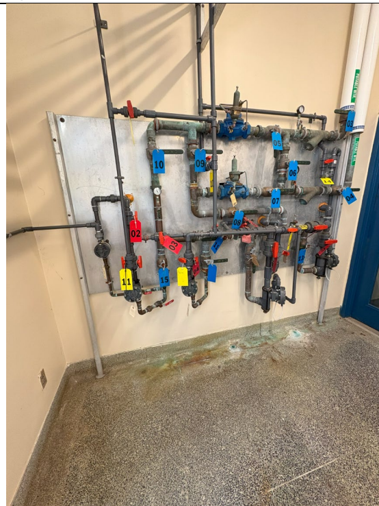
Figure 88: Chlorine Zebra Mussel Control
