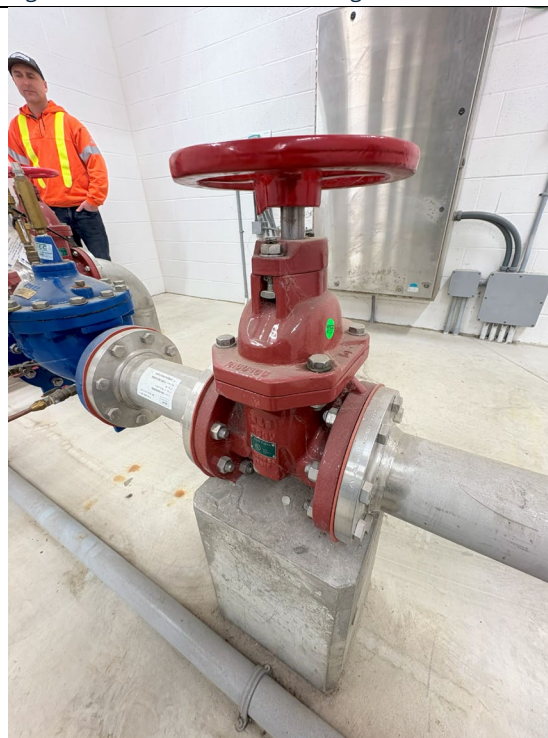
Figure 289: Discharge Gate Valve on PRV
