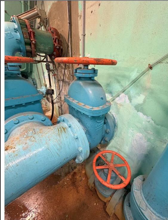
Figure 563: Gate Valve Discharge of Pump #4
