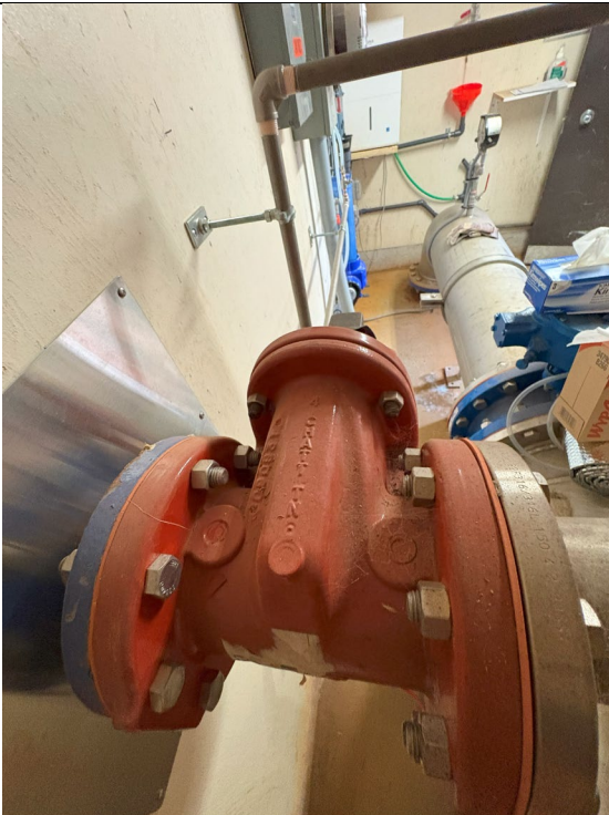
Figure 503: Gate Valve
