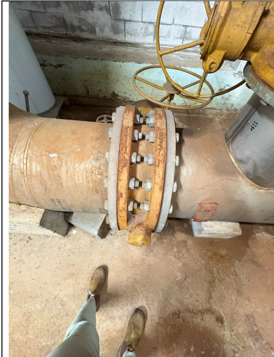
Figure 346: Pump #1 Butterfly Valve
