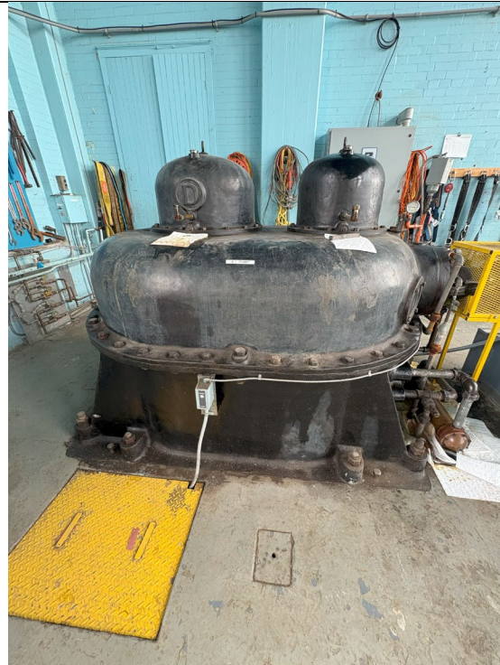
Figure 422: Gear Increaser on Pump #1
