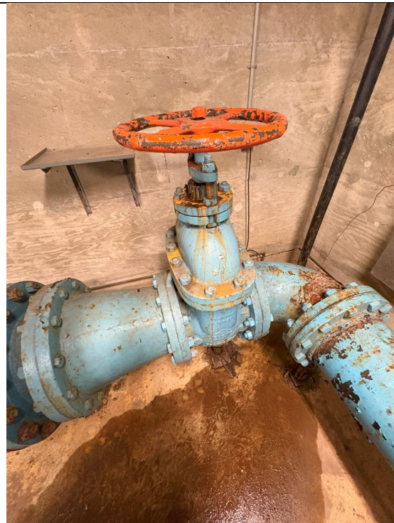
Figure 160: Gate Valve in Southwest Corner of Station
