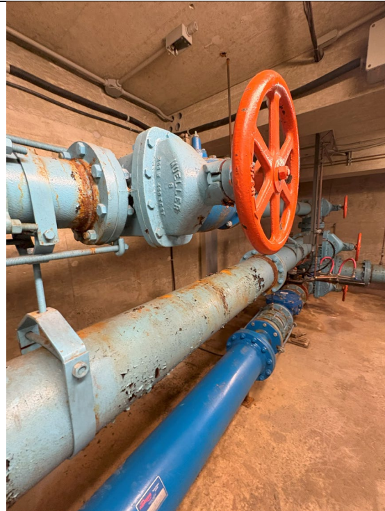
Figure 164: Gate Valve on Pressure Reducing Valve
