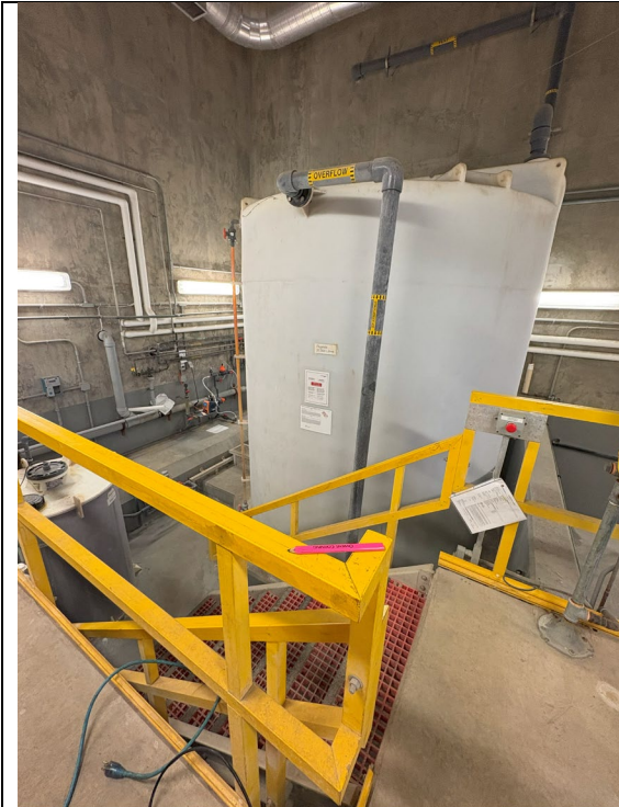
Figure 17: 25,000L Fluoride Storage Tank
