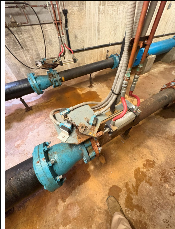
Figure 195: Reducer on Pump #2
