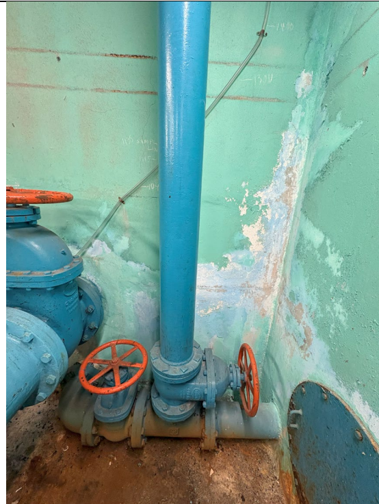
Figure 564: 4" Gate Valve
