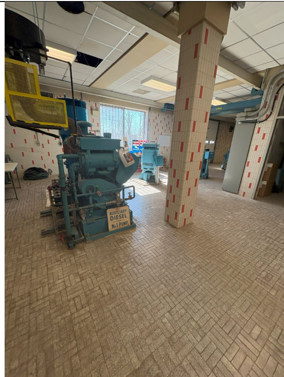
Figure 68: Pump #1 Diesel Motor
