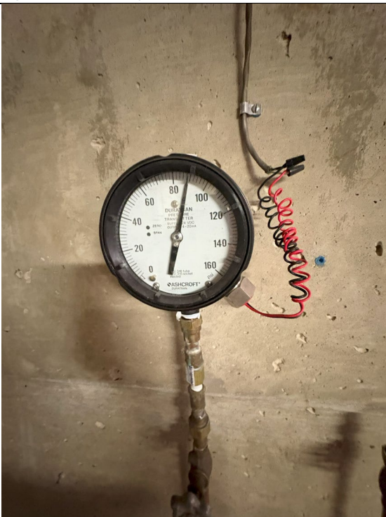
Figure 169: Discharge Pressure Gauge Zone 2
