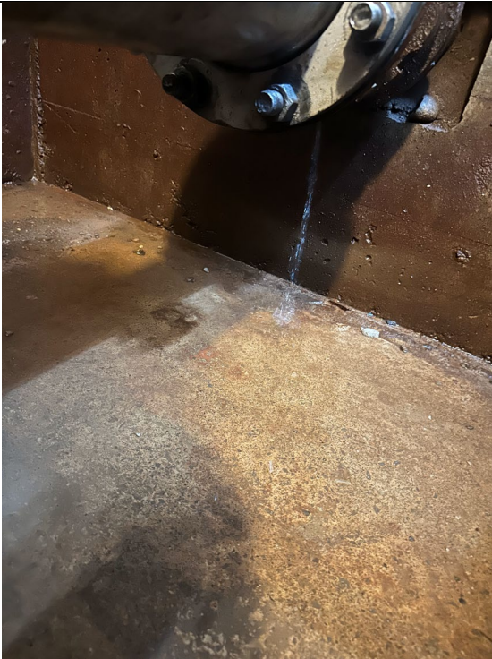
Figure 441: Defect in Drainpipe, Constantly Leaking
