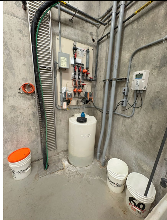
Figure 134: Dechlorination Station
