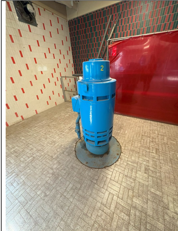
Figure 65: Backwash Electric Motor #2
