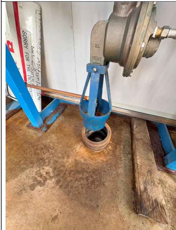
Figure 633: Backflow Preventer
