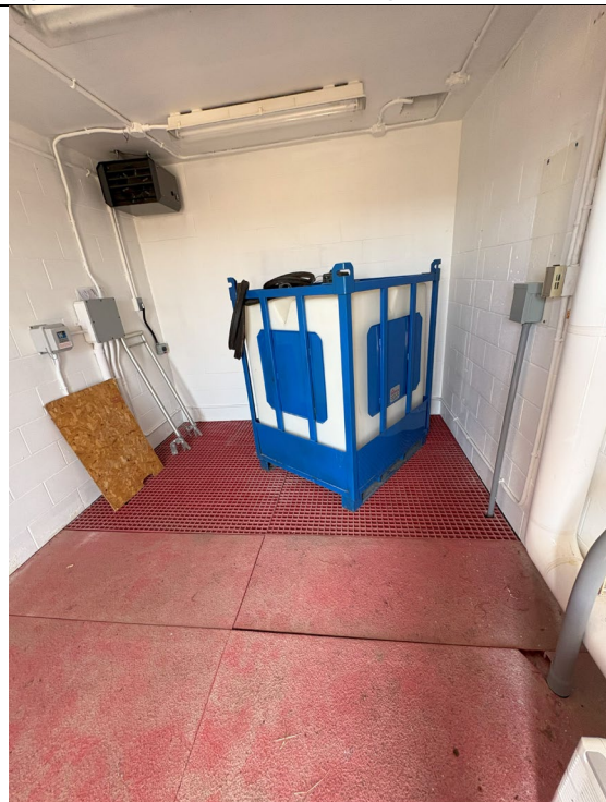
Figure 598: Chlorine Tank in Bricked Building
