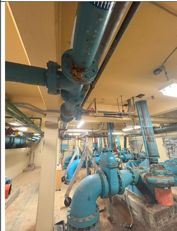
Figure 79: Plant Service Water Piping Corrosion
