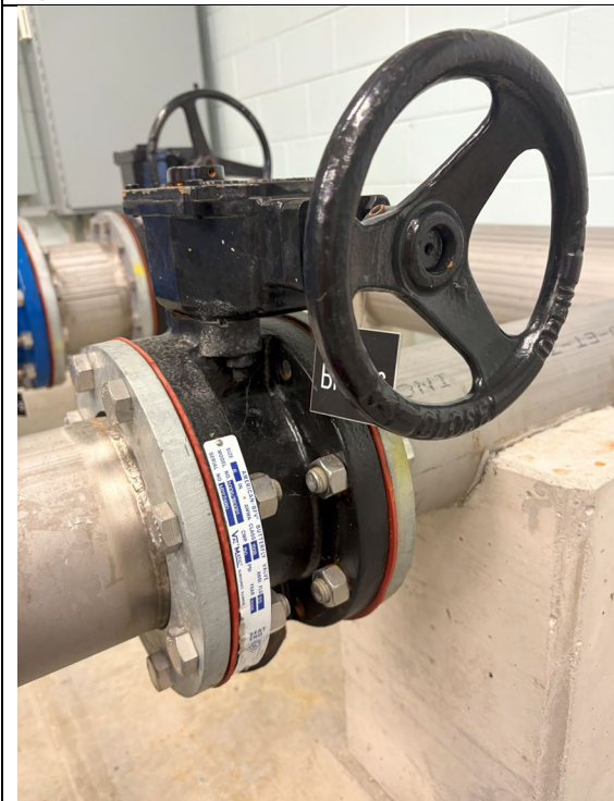
Figure 233: Butterfly Valve #6
