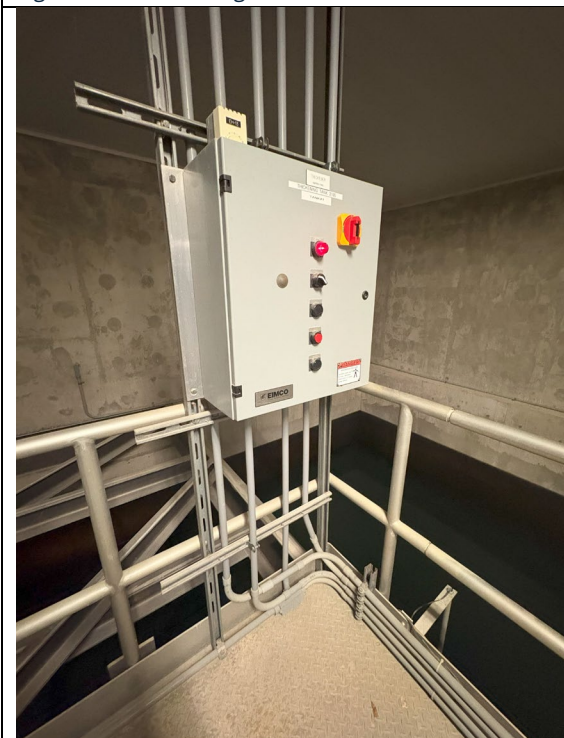
Figure 139: Thickening Tank #1 Controls
