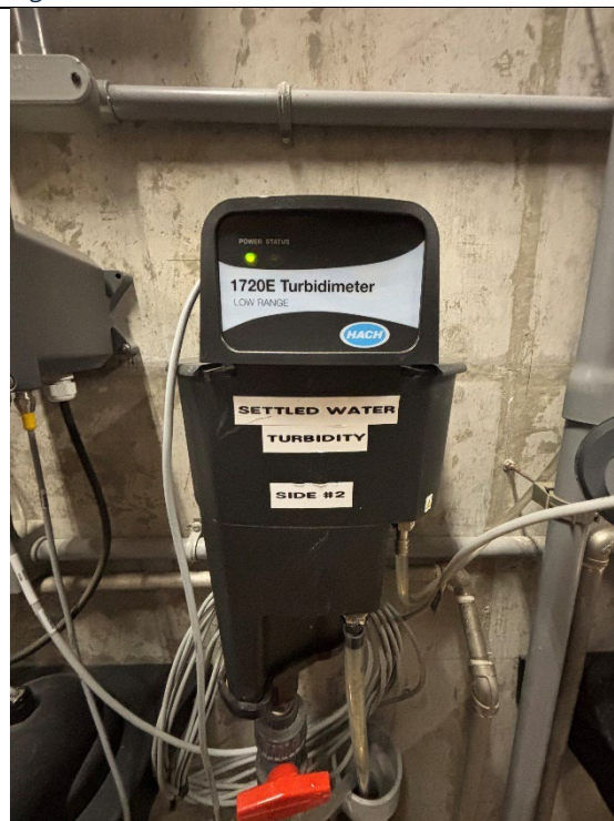
Figure 124: Pilot Plant Turbidity Meter
