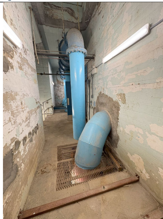
Figure 4: Piping Between Wet Well and Low Lift Pumps
