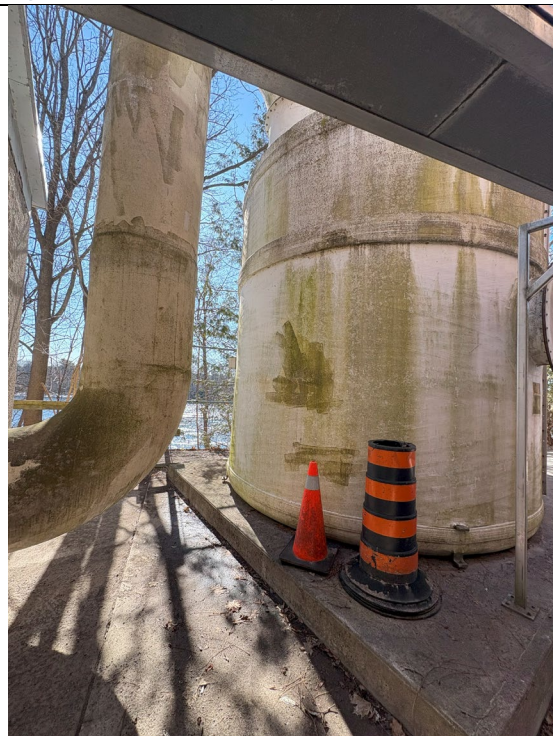
Figure 84: Chlorine Scrubber
