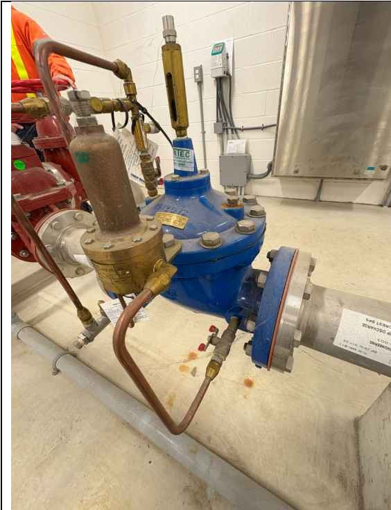
Figure 290: Pressure Reducing Valve
