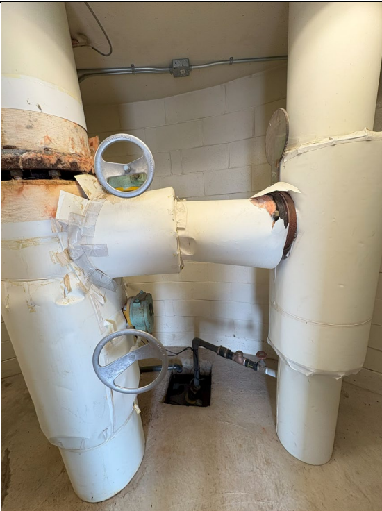
Figure 534: Two Butterfly Valves on 12" Feed
