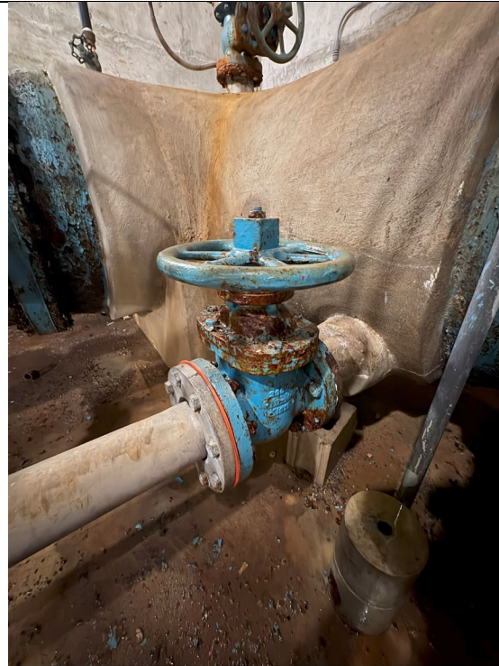
Figure 612: Gate Valve
