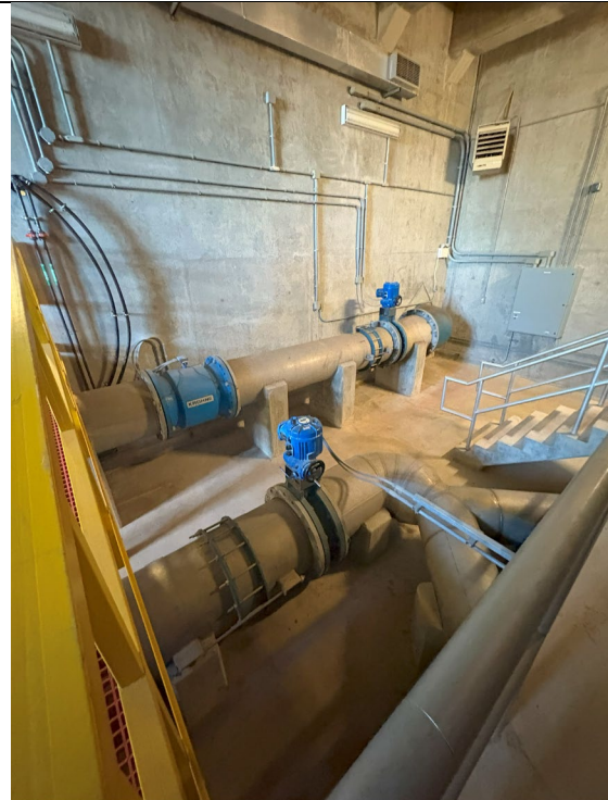
Figure 14: Post Coagulation Injection Mixers
