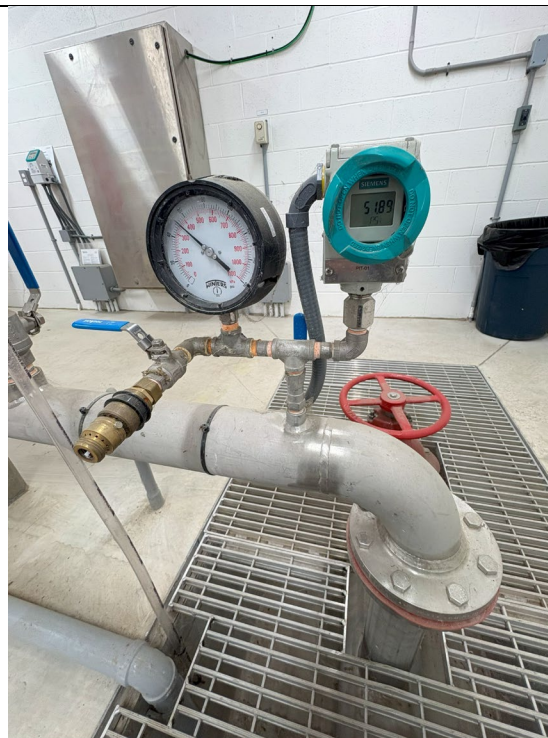
Figure 287: Suction Pressure Gauge Zone 2
