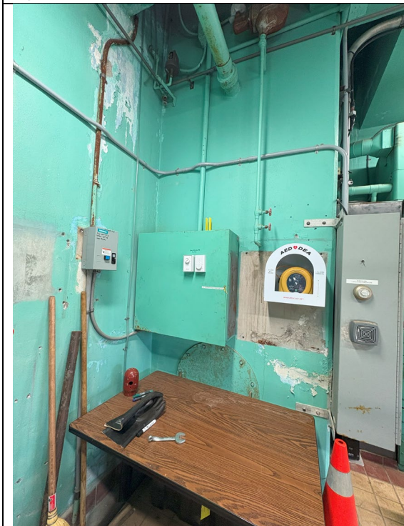
Figure 545: Peeling Paint
