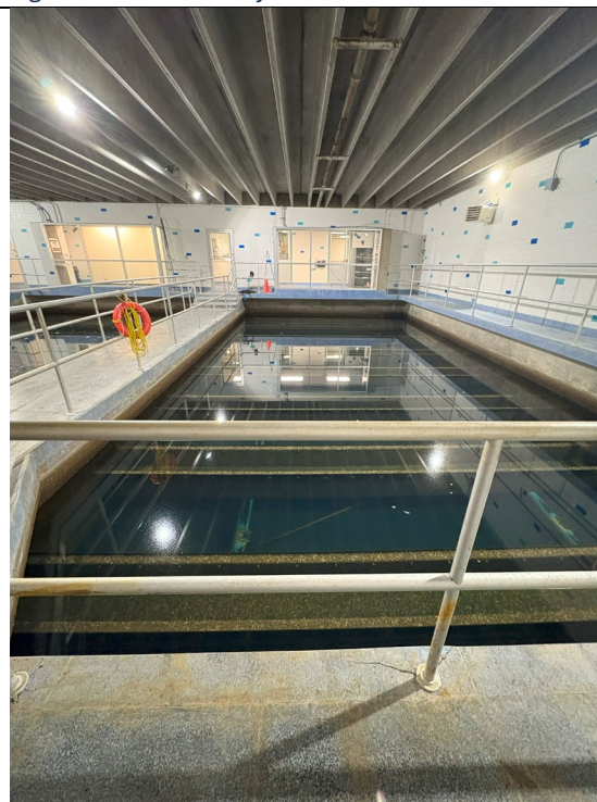
Figure 40: Filter Bed #11
