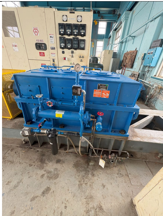
Figure 407: Generator #3 Gearbox, Recently Rebuilt
