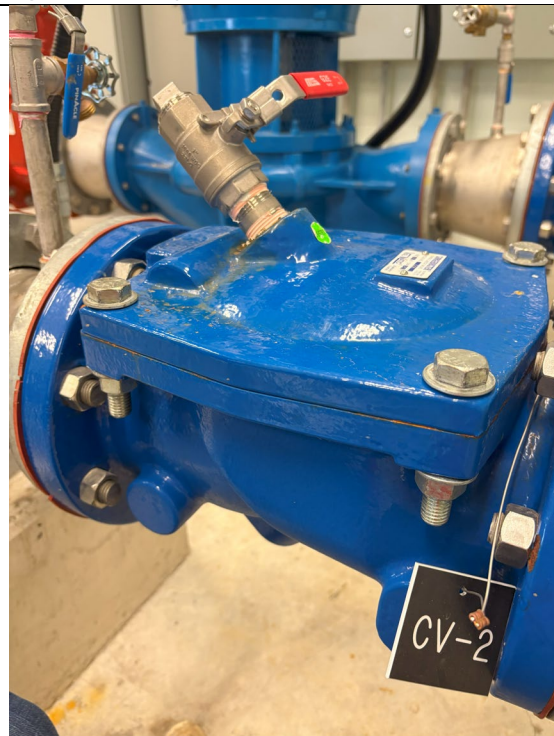
Figure 234: Check Valve #2
