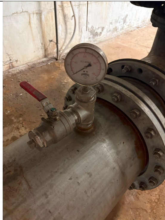
Figure 351: Suction Pressure Gauge
