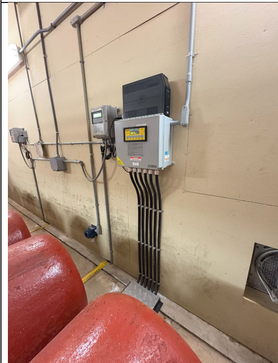
Figure 83: Gas Cylinders Safety System
