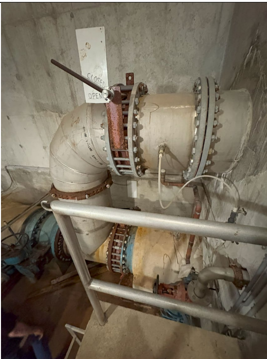
Figure 601: Butterfly Valve
