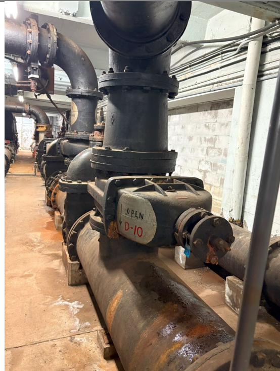
Figure 370: Pump #5 16" Discharge Gate Valve (D10)
