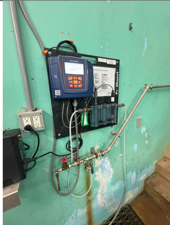
Figure 588: Chlorine Monitor
