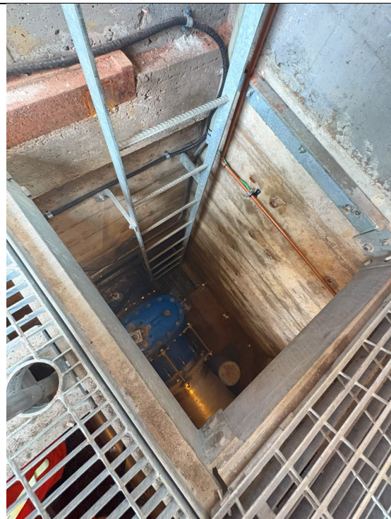
Figure 440: Access Ladder to Process Piping
