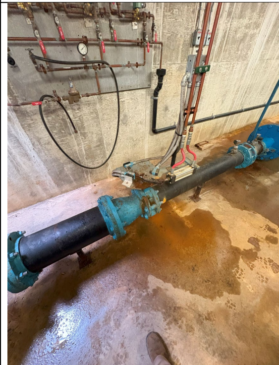
Figure 197: Reducer on Pump #3
