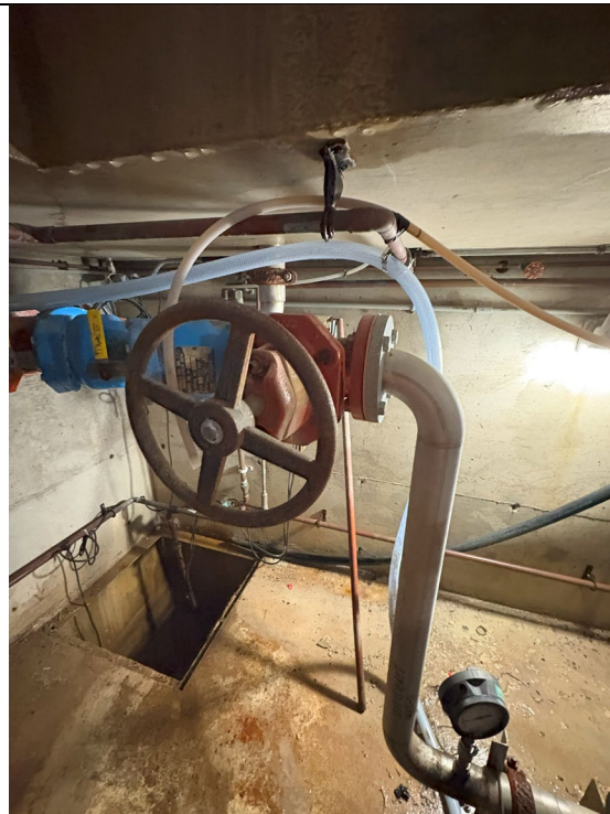
Figure 616: Gate Valve and Sump Pump
