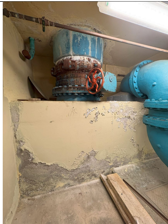
Figure 80: High Lift Pump Piping Corrosion
