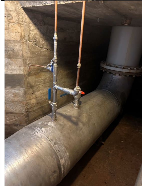
Figure 445: 500mm Stainless Steel Pipe, Tower Intake
