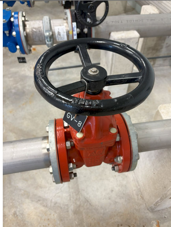
Figure 224: Gate Valve #8
