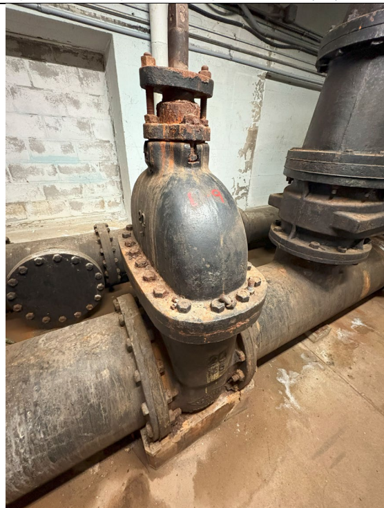
Figure 368: Zone 1 20" Discharge Gate Valve
