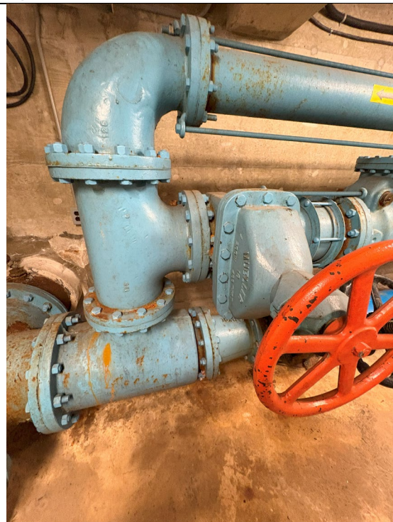
Figure 162: Gate Valve
