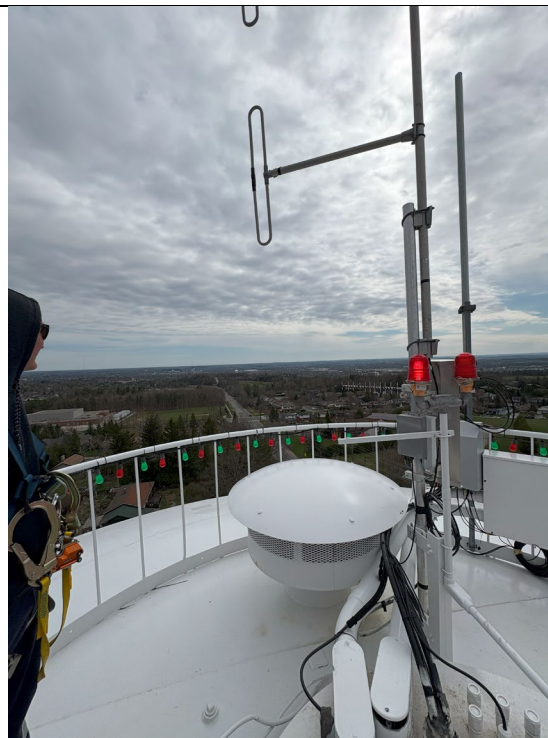
Figure 486: Breather Vent at Top
