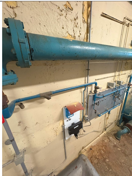
Figure 58: Plant #2 Pipe Gallery Paint Peeling
