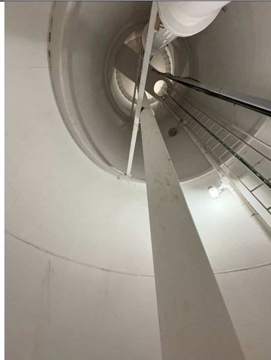
Figure 474: Water Tower Process Piping
