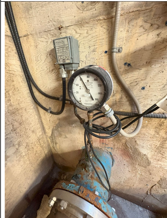
Figure 312: Suction Pressure Gauge
