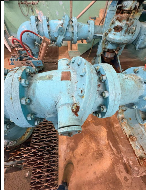
Figure 555: Check Valve on Pump #2
