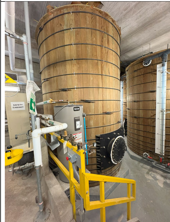
Figure 19: 3x 18,000L Coagulation Tank
