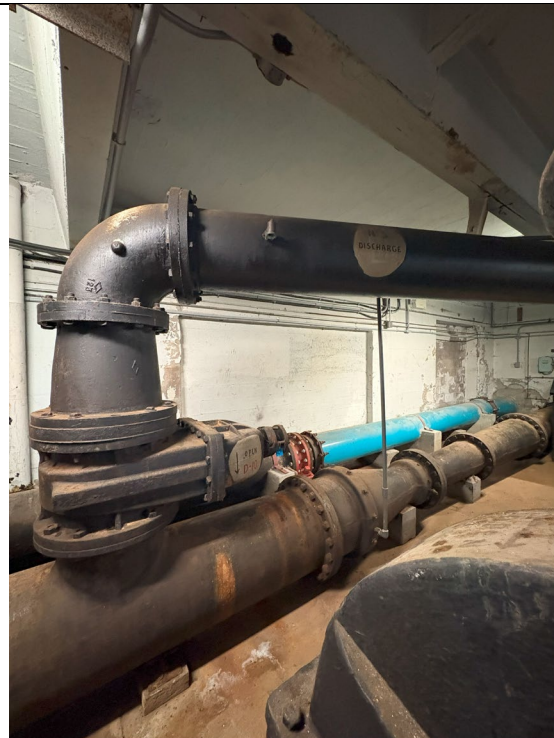
Figure 386: Pump #5 Discharge Piped
