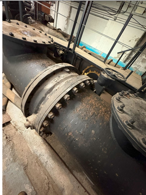
Figure 380: 30" Butterfly Valve
