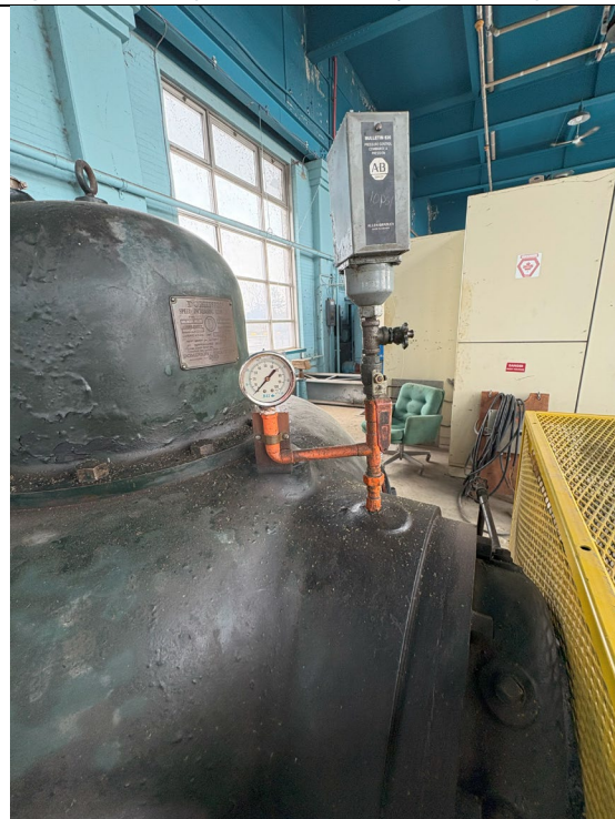
Figure 400: Pressure Gauge on Pump #4
