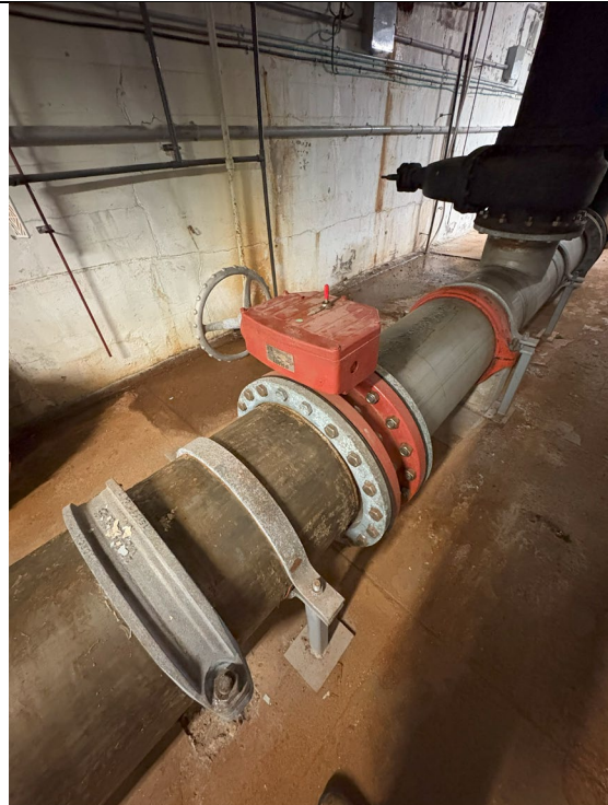
Figure 354: 20" Butterfly Valve
