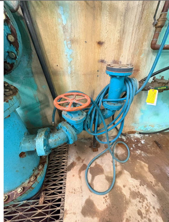
Figure 579: 4" Gate Valve
