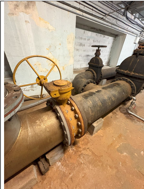
Figure 358: Butterfly Valve
