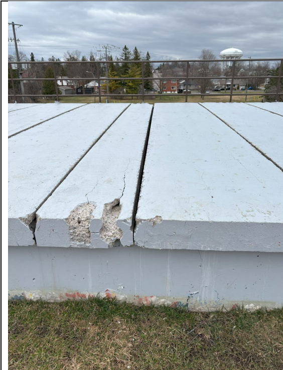
Figure 539: Deteriorated Concrete Roof
