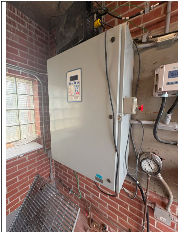
Figure 449: SCADA Cabinet
