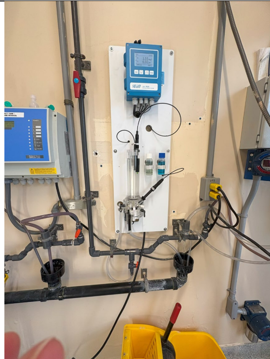
Figure 86: Post Chlorine Swan Disinfection Monitor
