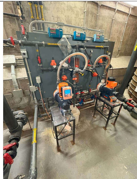
Figure 20: Coagulation Pumps Piping & Controls
