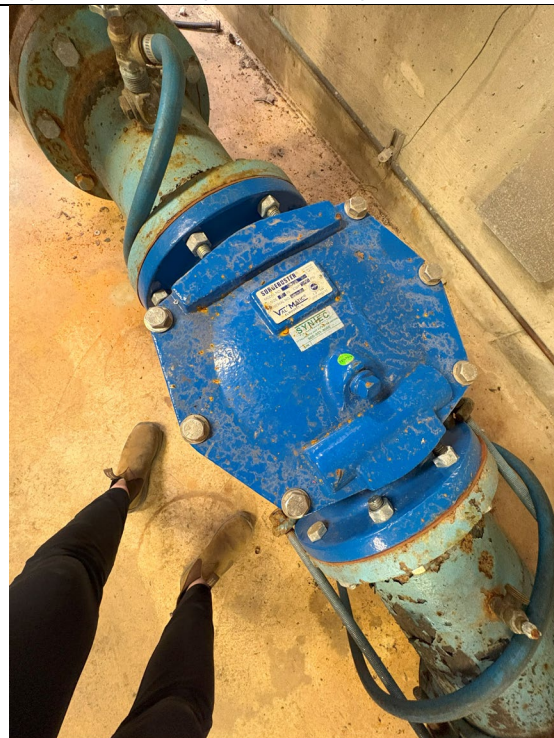
Figure 158: Swing Check Valve on Pump #3
