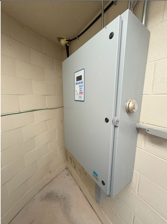
Figure 536: SCADA Control Box
