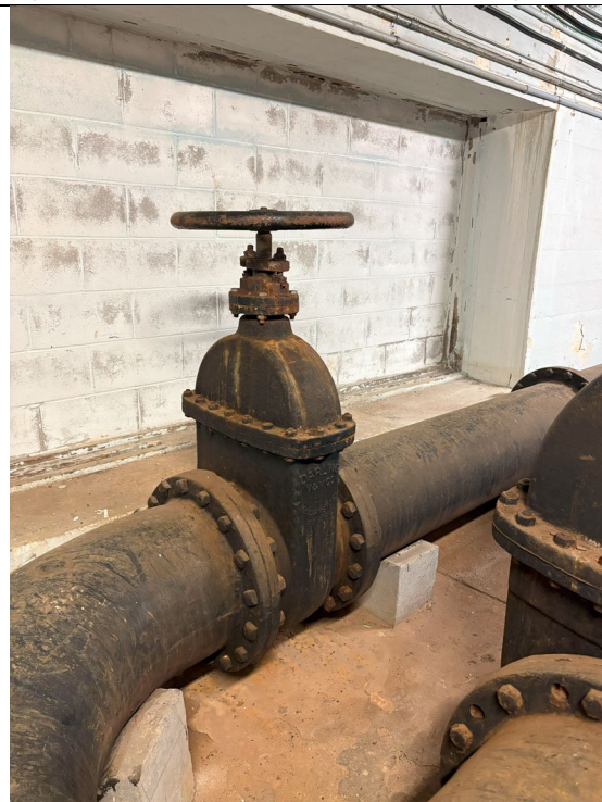
Figure 361: Zone 1 Discharge Gate Valve
