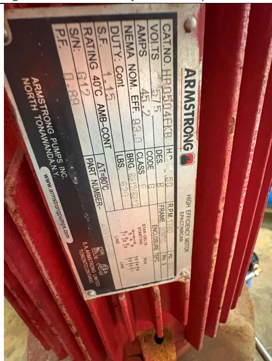
Figure 153: Label on Pump #2
