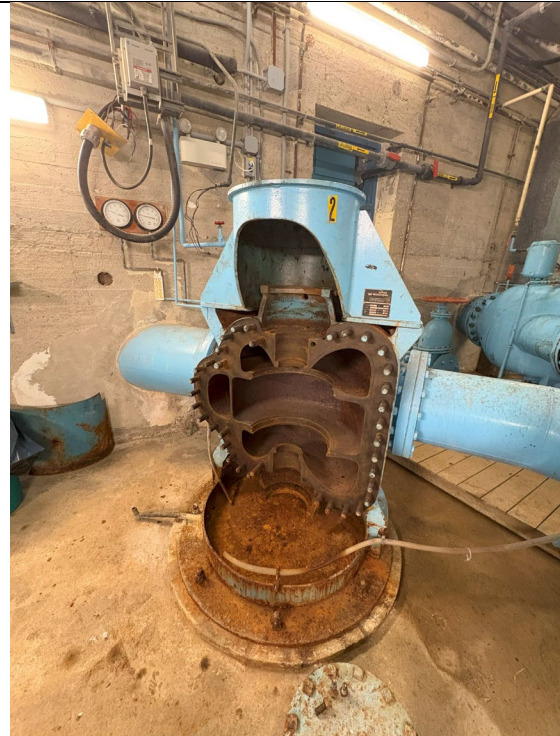
Figure 6: Electric Pump #2 Being Repaired
