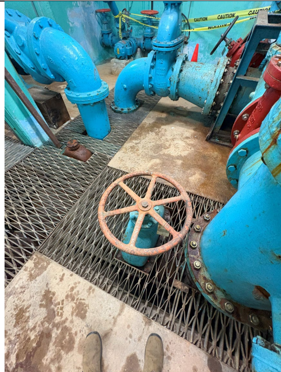
Figure 580: 18" Gate Valve
