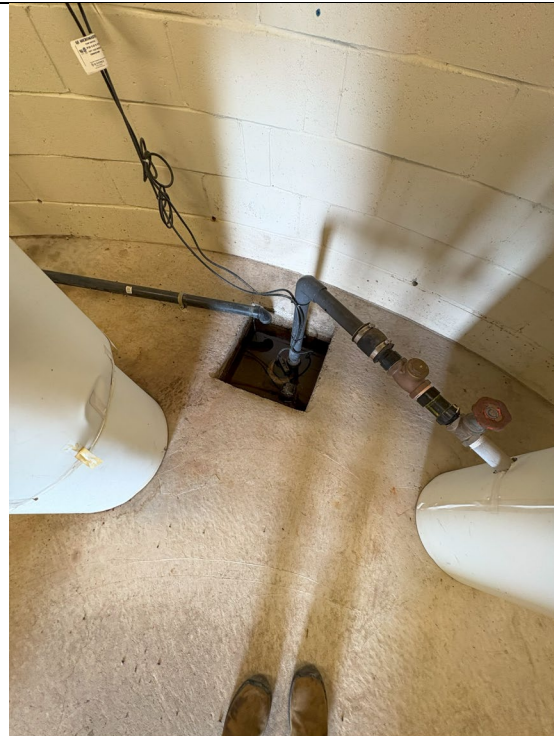
Figure 535: Sump Pump
