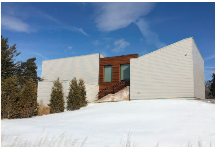
Peterborough Museum & Archives construction completed—west elevation, January 2017.
