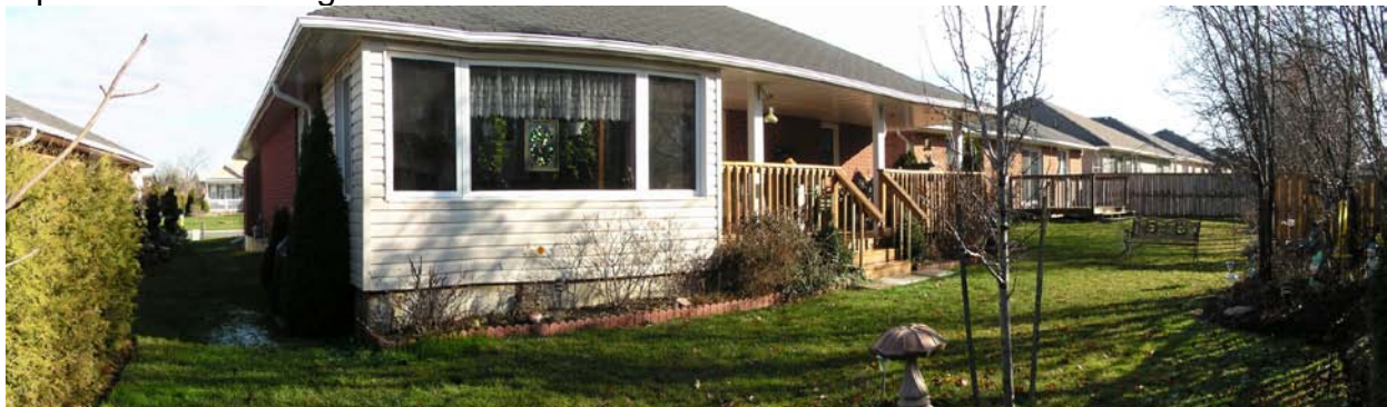
Addition to the rear of 1587 Ravenwood Drive
